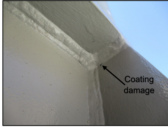
72. Chipped outer coating at anchor stud #1
