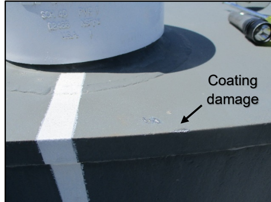
86. Coating damage at edge NE quadrant
