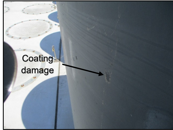
89a. Coating damage overpack SW quadrant (close-up)
