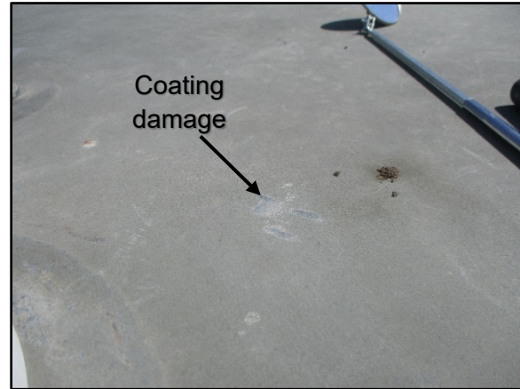
32. SW lid coating damage
