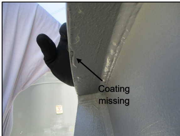
58. Missing outer coating between anchor studs #10 & #7
