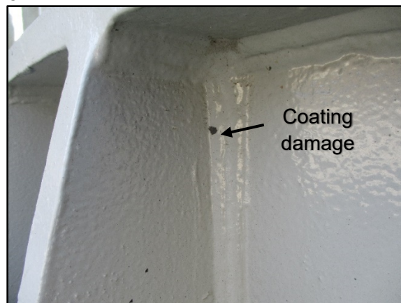
49. Area adjacent to anchor stud #16 outer coating chip
