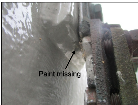
18. 90° ground strap underside
