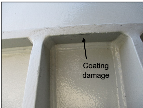
54. Anchor stud #12 outer coating chip
