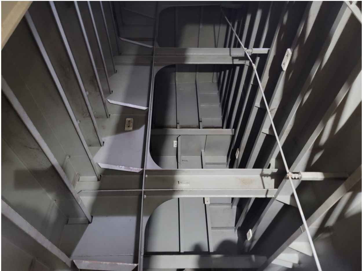
Photograph 2-2 Tank 9P Internal Support Structure
