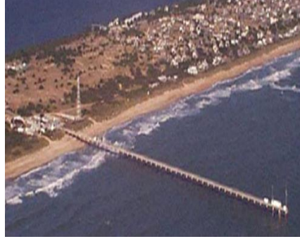
Figure 5-24 USACE ERDC CHL Field Research Facility [54]
