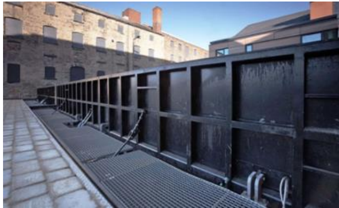
Figure A-4 Hydraulically Activated Barrier [70]
