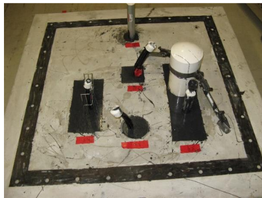
Figure 5-18 A Test Deck with Penetration Seal Installed [5]
