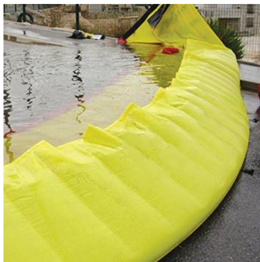
Figure 4-7 AquaDam® Used in Fort Calhoun Station During the 2011 Flood Event [43]
