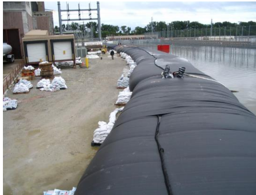
Figure 4-7 AquaDam® Used in Fort Calhoun Station During the 2011 Flood Event [43]
