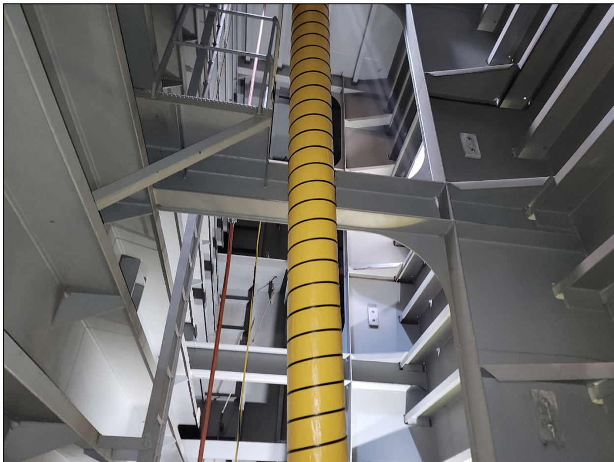
Photograph 2-1 Access Ladder, Platforms, and Ventilation Trunk
