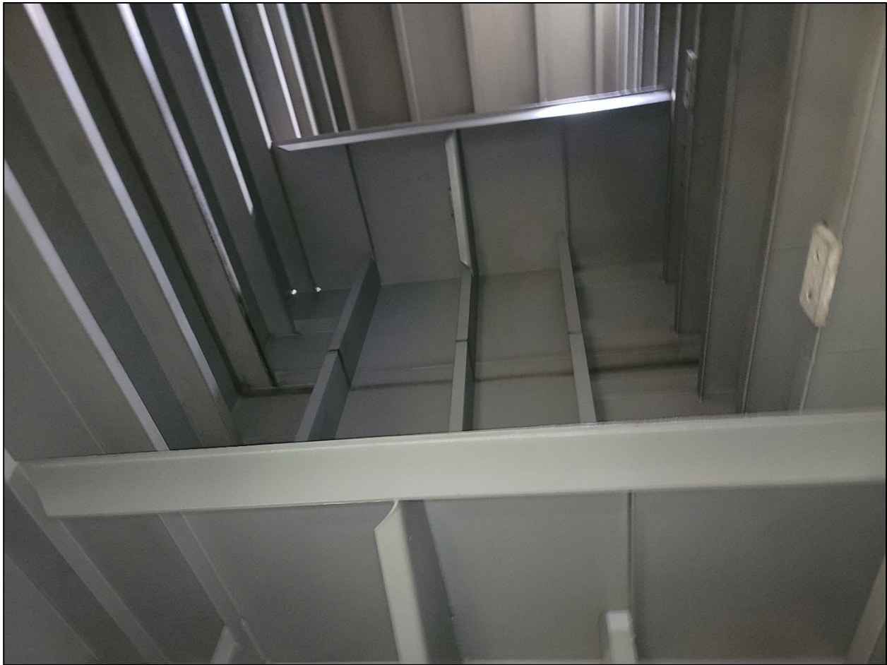
Photograph 2-2 Internal Support Structure
