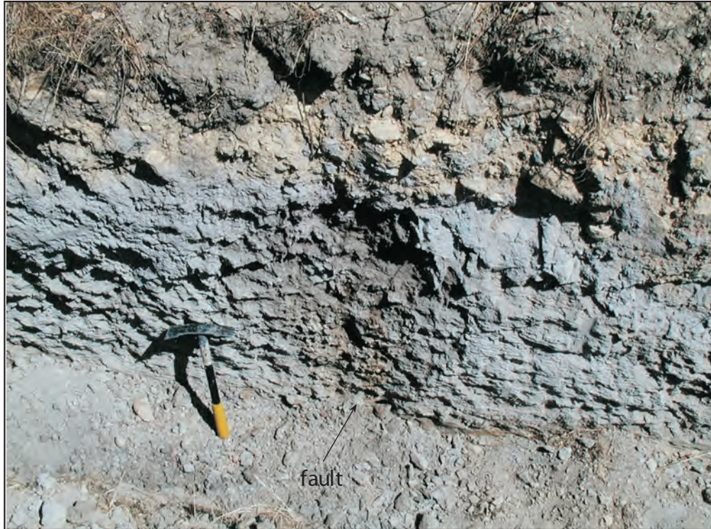
Friable sandstone ( Tof_{b-2a} ) in trench T-1. The friable sandstone generally is weakly bedded and jointed. A small near-vertical fault is indicated by oxidized clay stringers in the sandstone. Photo roll JLB-3.
