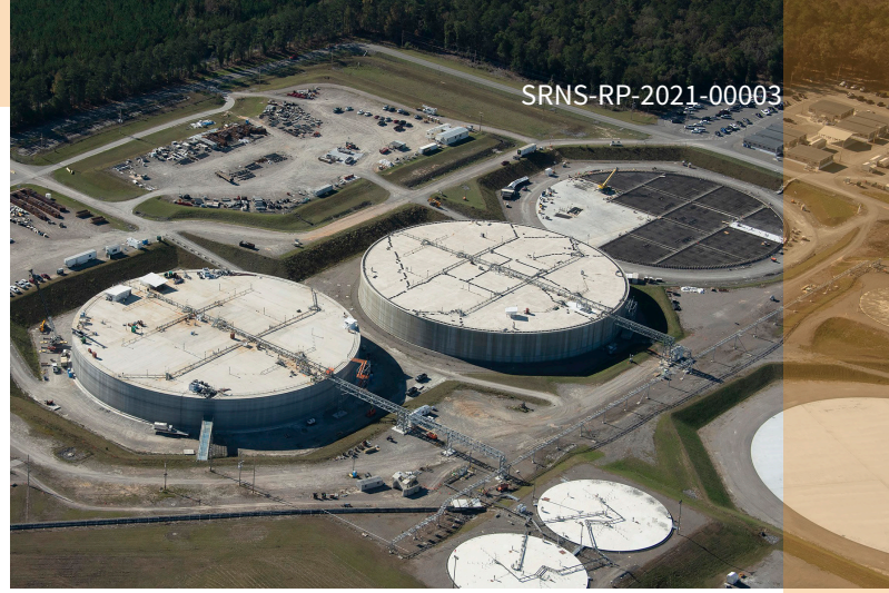
Saltstone Disposal Units 8 and 9, under construction, will be the newest mega-tanks to permanently store saltstone at the Savannah River Site.
