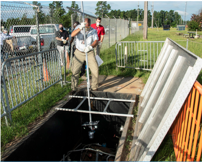
Vacuum equipment (top photo) was used to remove water from the tank, exposing a layer of sludge containing silver. A worker (bottom photo) lowers the camera to inspect the inside of the tank.
