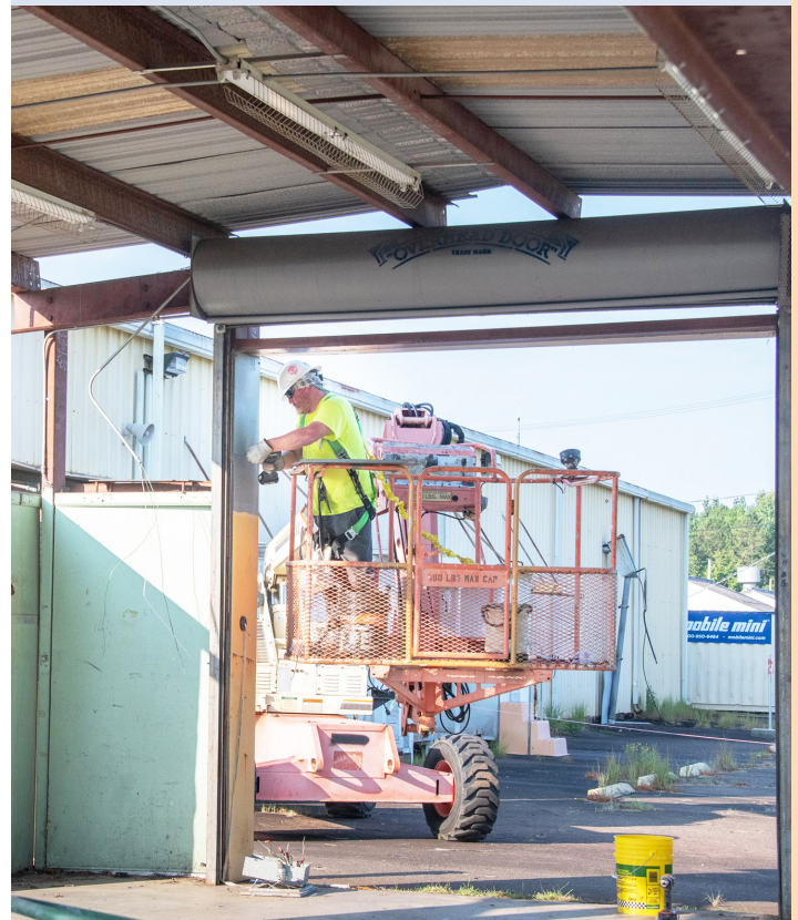
The Site donated unused metal buildings, saving disposition costs while benefiting the community.
