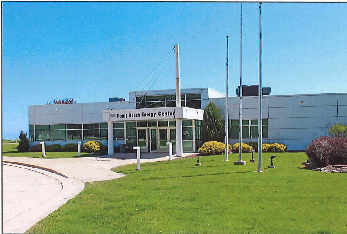
Figure 21. Energy Center, View East
