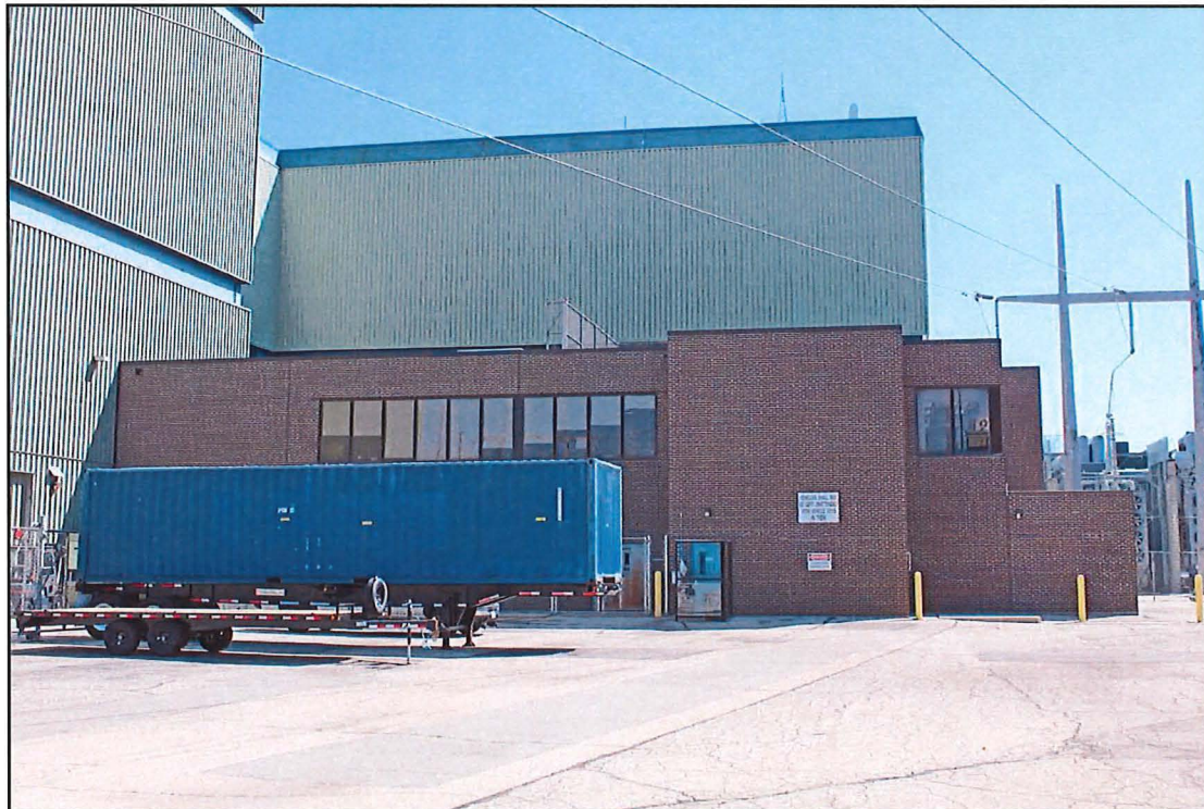
Figure 16. South Service Building, View East
