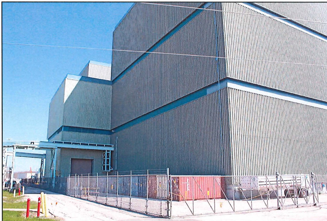
Figure 10. Reactor Containment Building, View Northeast
