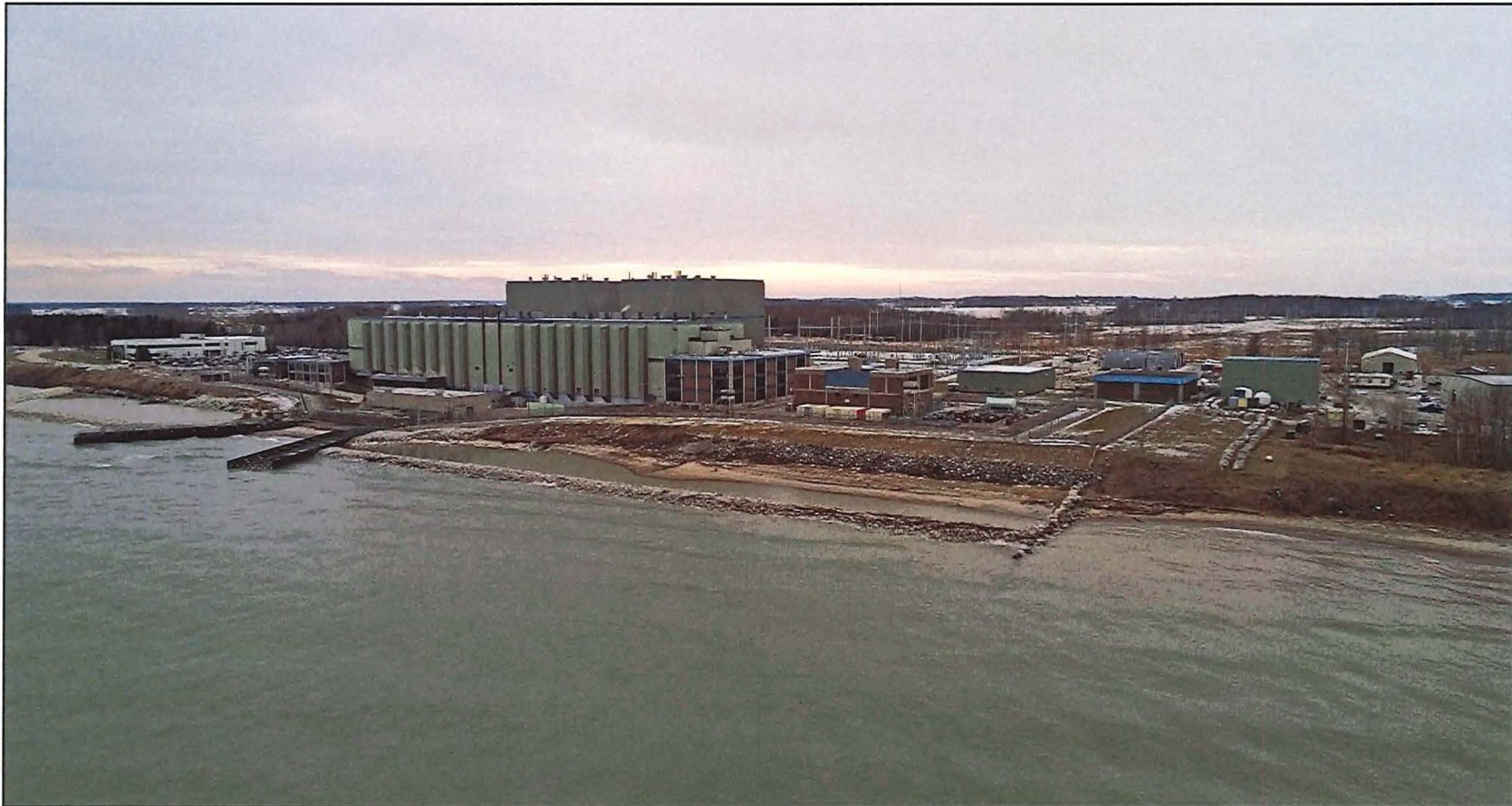
Figure 4. December 2019 Drone Photograph of Property from Lake Michigan, View Southwest Source: NextEra Energy
