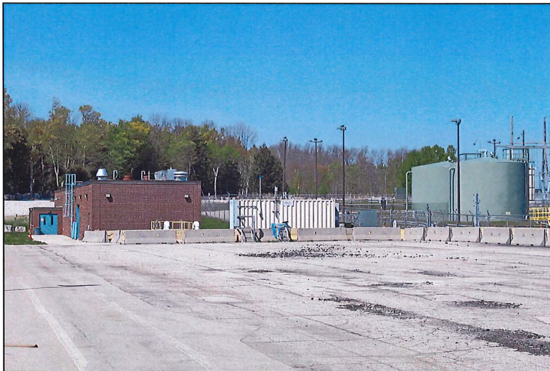
Figure 18. Sewage Treatment Plant, View West
