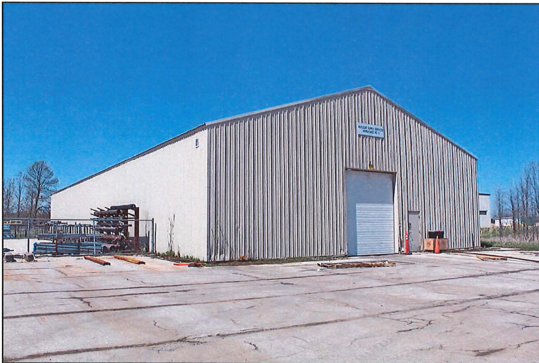
Figure 26. Warehouse 5, View West
