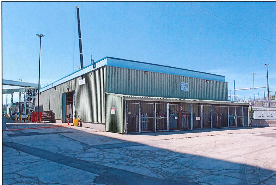
Figure 14. Warehouse 2, View Southwest
