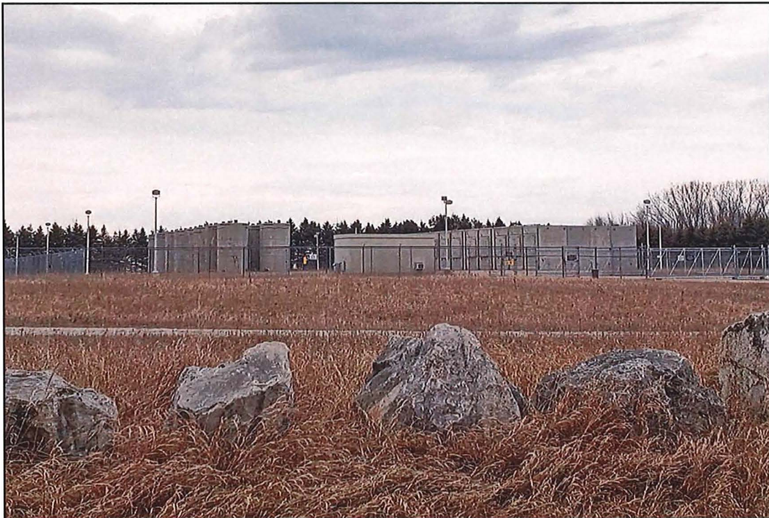
Figure 32. ISFSI Facility, View Northeast
