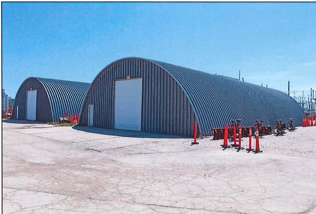
Figure 30. Quonset Huts, View Southeast
