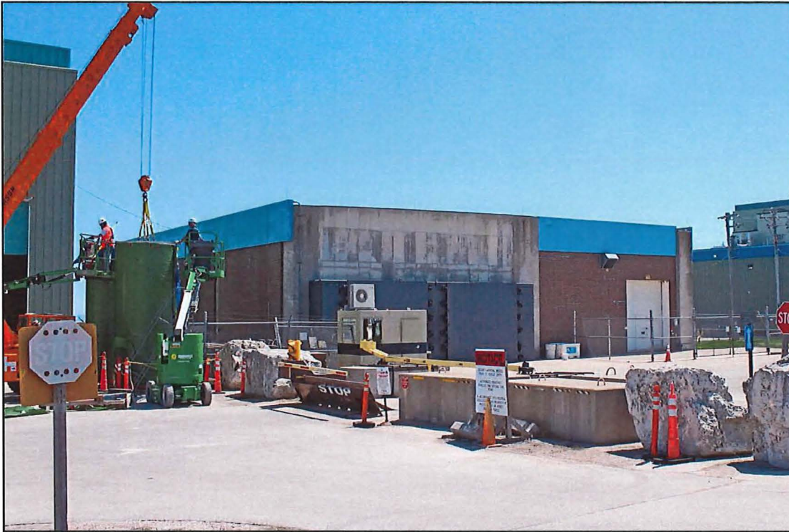
Figure 29. Flex Building/Warehouse, View Southeast
