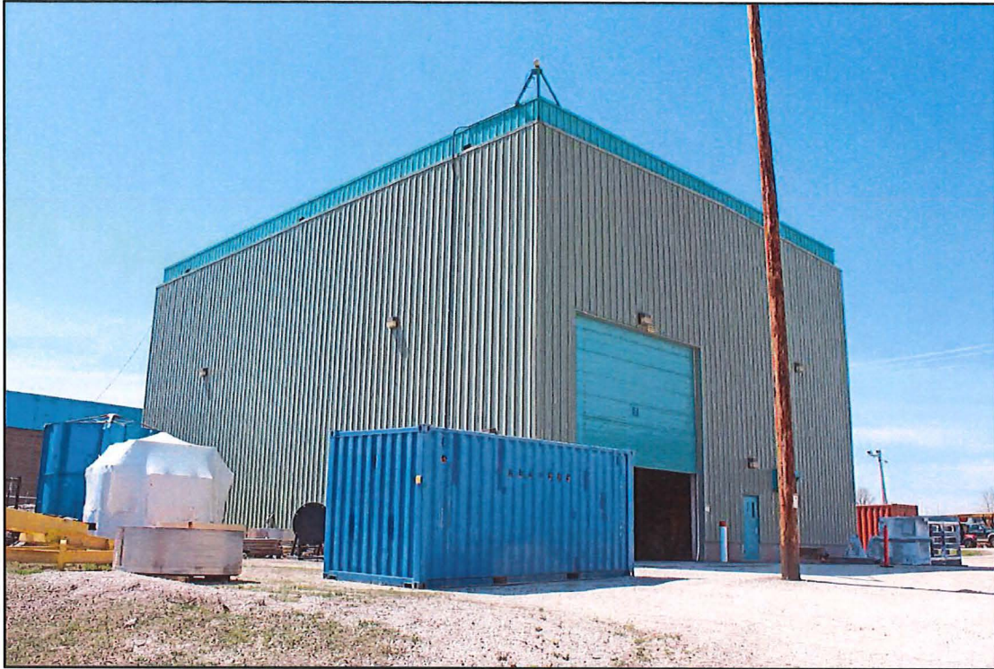
Figure 25. Transporter Building, View Northwest
