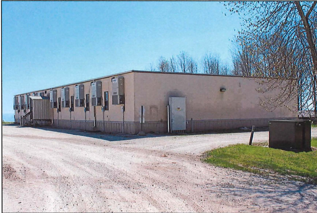
Figure 23. Trailer 10, View Southeast
