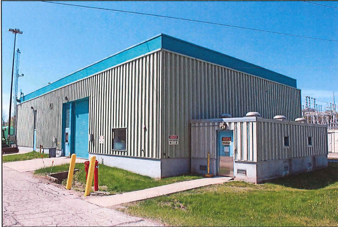
Figure 13. Warehouse 1, View South
