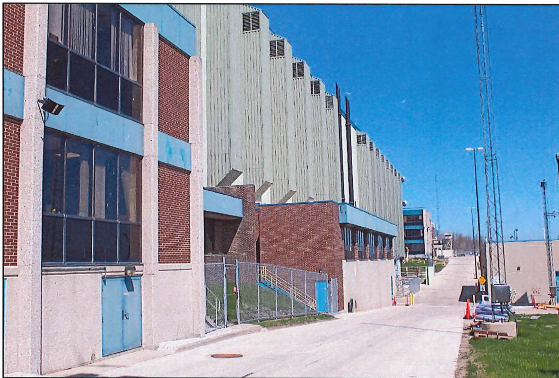
Figure 8. Turbine Building, View North
