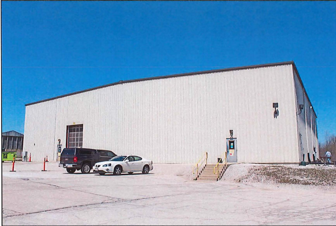
Figure 27. Warehouse 6, View North
