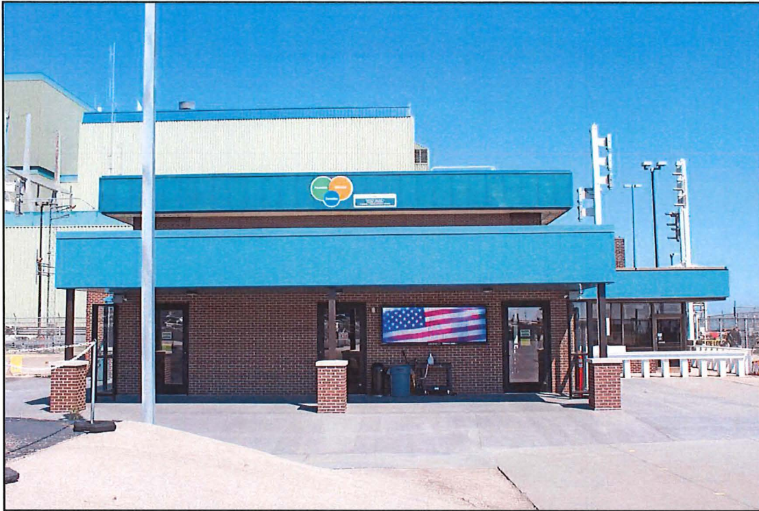
Figure 17. Security Gate House, View North
