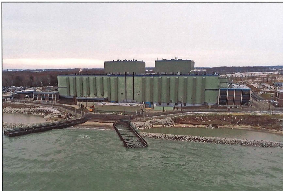
Figure 6. December 2019 Drone Photograph of Turbine Building, View West Source: NextEra Energy
