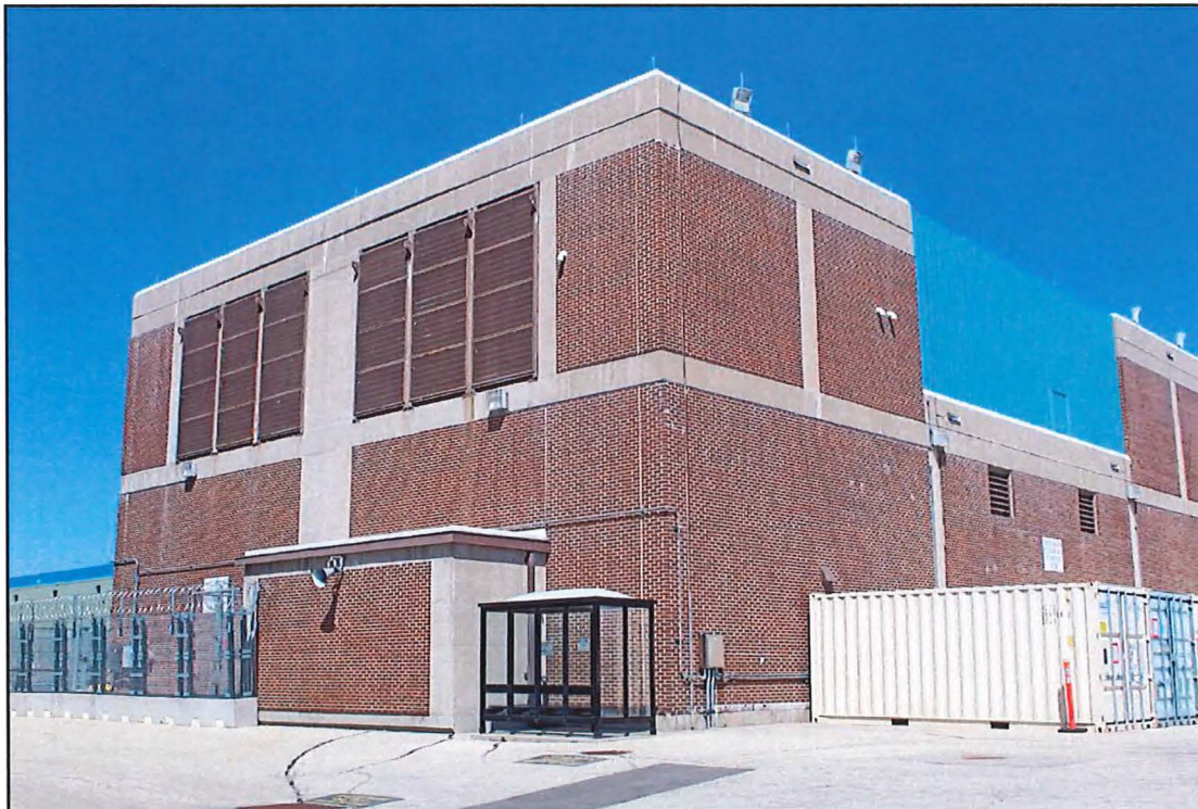
Figure 12. Emergency Diesel Generator Building, View Northwest
