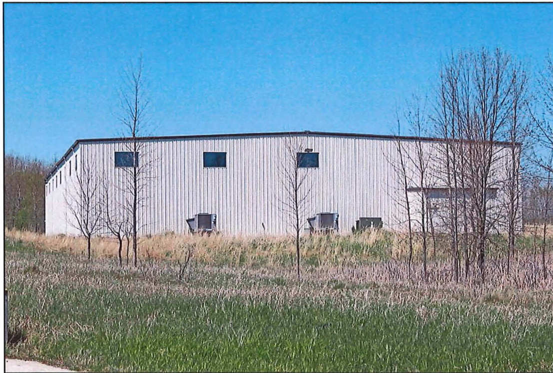
Figure 28. Warehouse 7, View West
