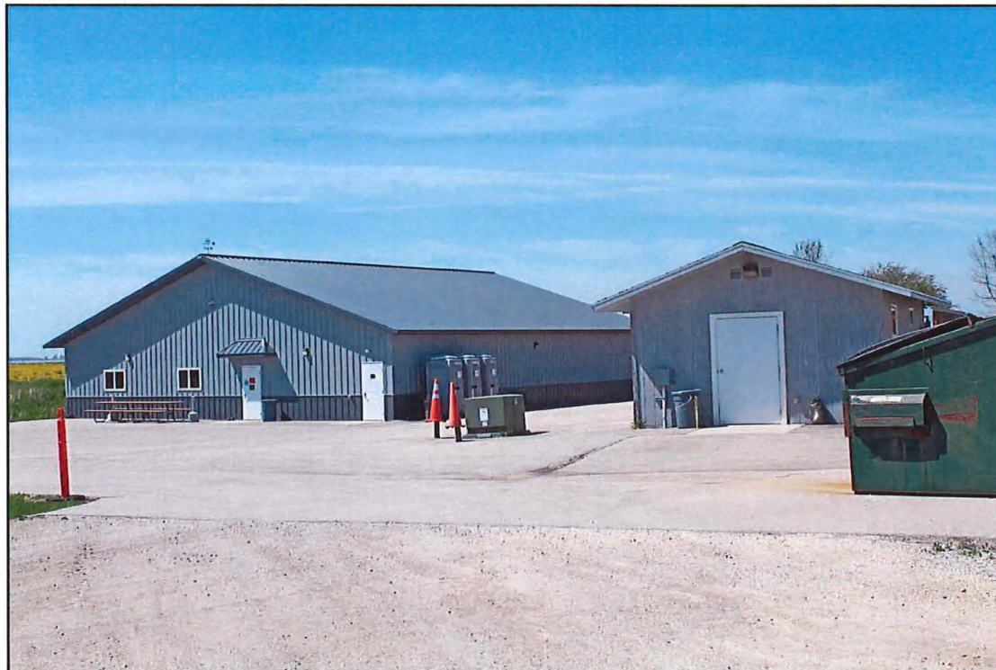
Figure 24. Shooting Ranger, View West
