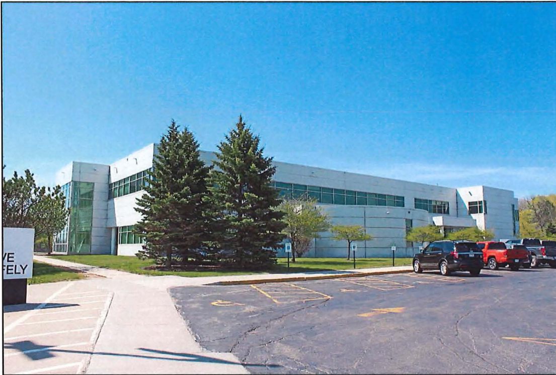
Figure 19. Training Building, View South
