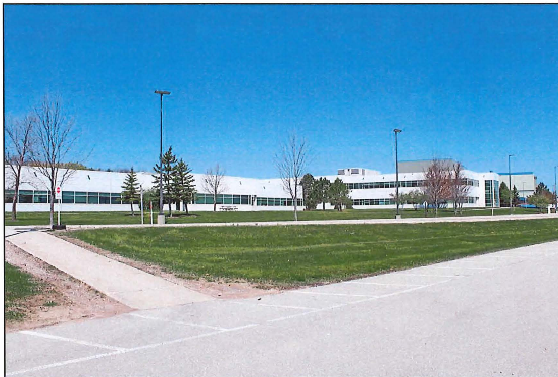
Figure 20. Engineering Building, View Northwest
