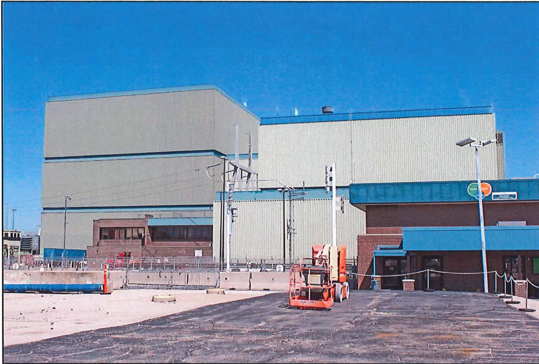
Figure 9. Unit 1 Reactor Containment Building (Left), View North
