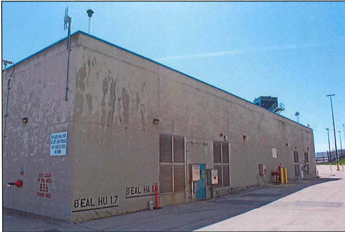
Figure 11. Circulating Water Pump House, View Southeast
