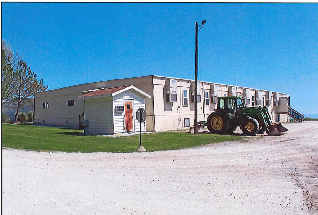
Figure 22. Trailer 9, View Northeast
