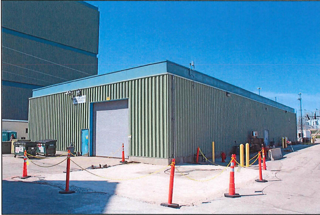
Figure 15. Warehouse 3, View Southwest
