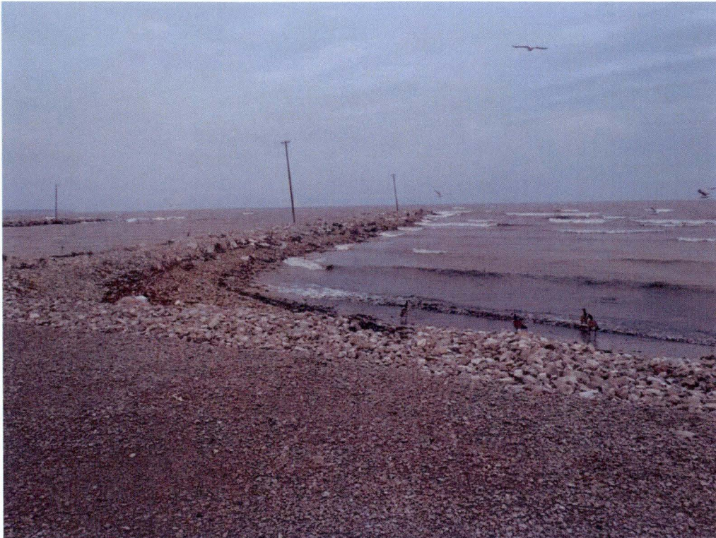
Photo – 10a: Looking east along South Groin (April 2011)
