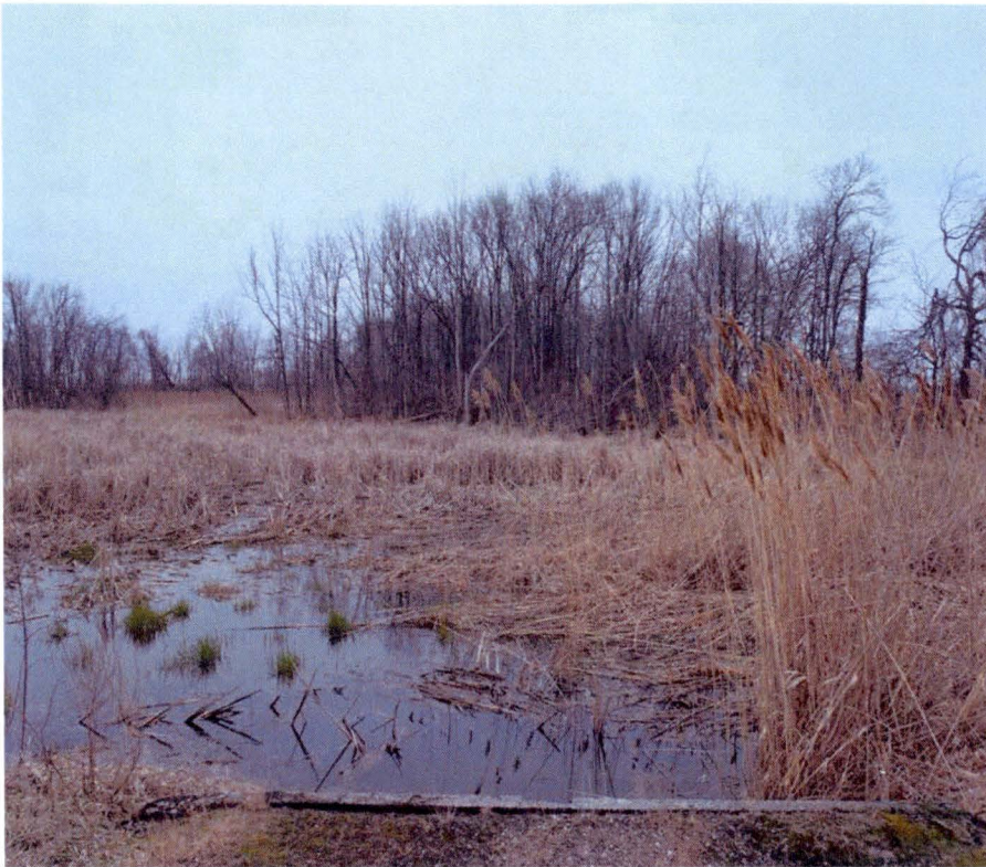
Photo – 14c: Upstream of existing culvert along Toll Road (April 2011)
