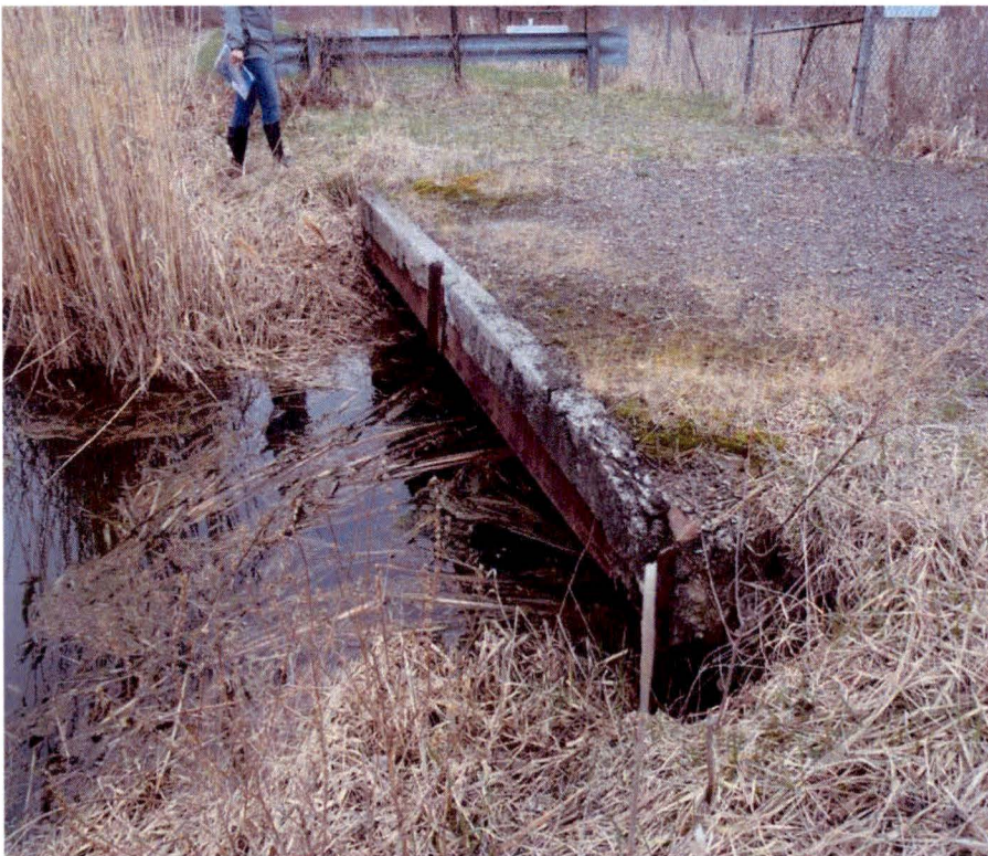
Photo – 14d: Upstream side of existing culvert along Toll Road (April 2011)
