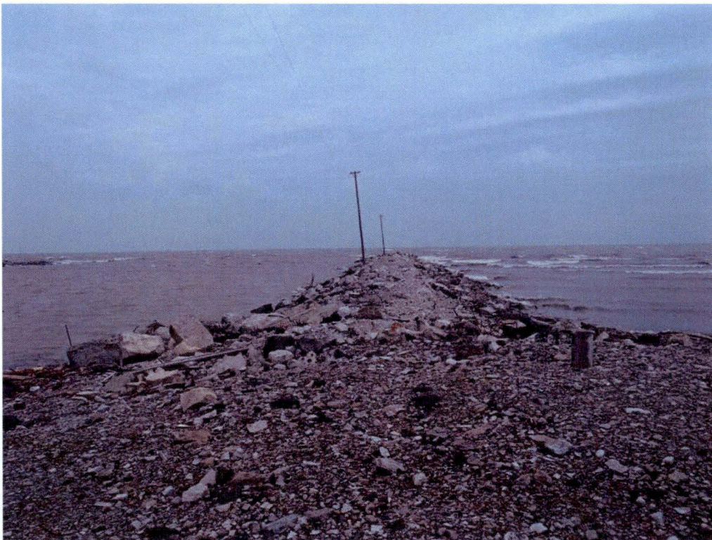
Photo – 10b: Looking east along South Groin (April 2011)
