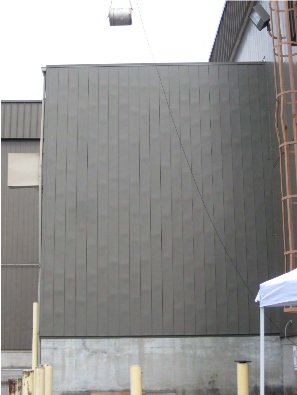
FIGURE B.1.3-1 – Test Unit Immediately Prior to HAC 30-Foot Side Drop
