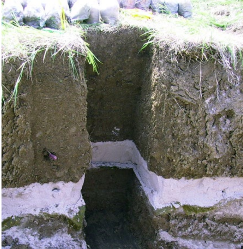
Figure 4.3-1: Analog Site: 8-Year-Old Engineered Cover in Omaha, NE
