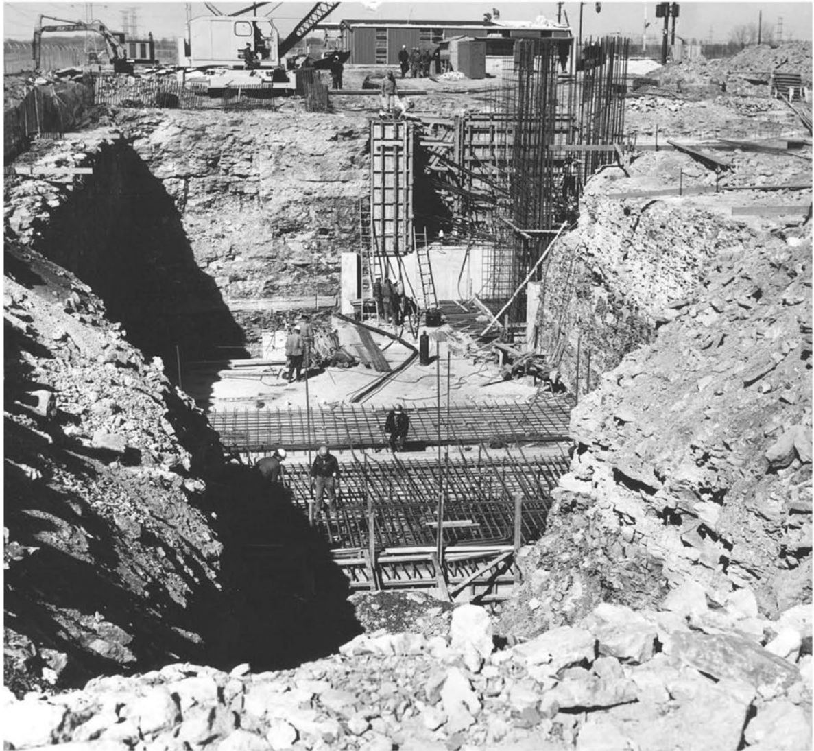
Figure 5-11. Excavation and Foundation Construction.
