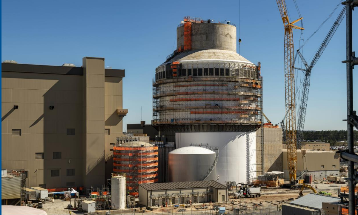
Vogtle Unit 3 Containment and Turbine Building
