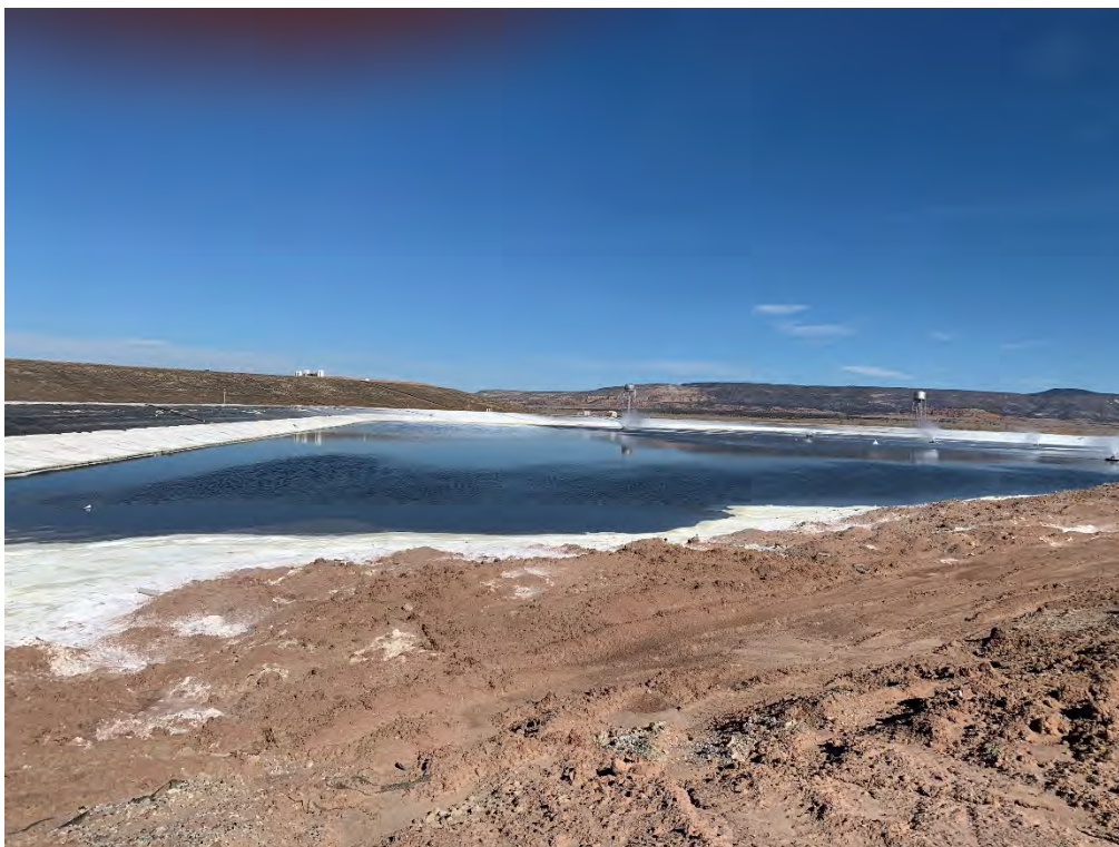
Photo 15: EP-1, precipitate buildup on slopes, operating at reduced capacity (looking north)
