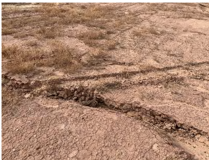
Photo 14: LTP, scour or damage to top surface interim cover
