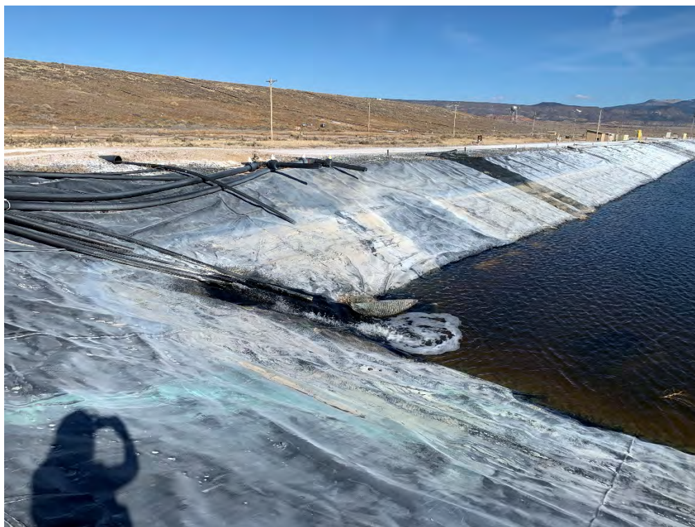
Photo 28: EP-2, general conditions, precipitate on northwest corner
