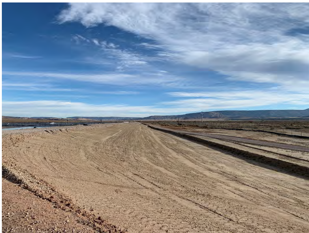
Photo 30: EP-3, general conditions of downstream slope after annual regrading
