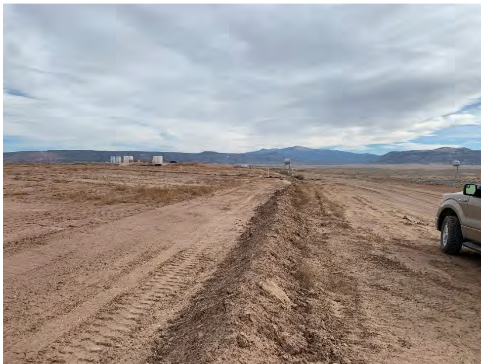
Photo 11: LTP, berm constructed to help divert stormwater on LTP top surface at the north side of road
