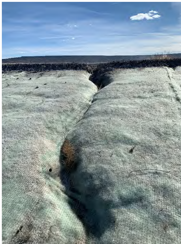
Photo 17: EP-1, erosion mat on north embankment, rilling present under mat
