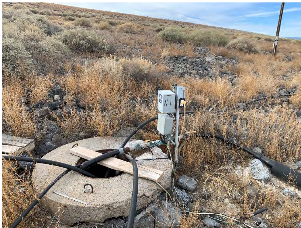
Photo 4: LTP, French drain/sump system at downstream toe of north side slope
