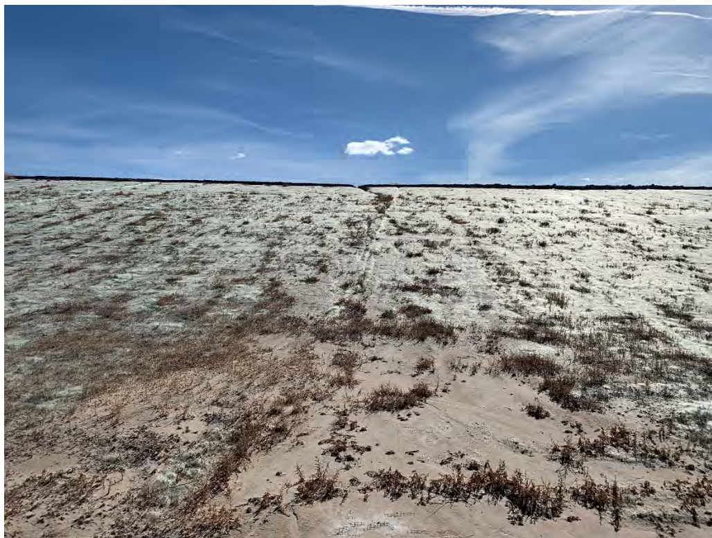
Photo 18: EP-1, erosion mat on the north embankment downslope
