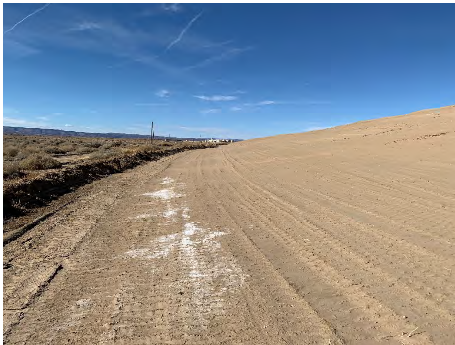
Photo 19: EP-1, downstream slopes of STP/EP-1 after annual regrading
