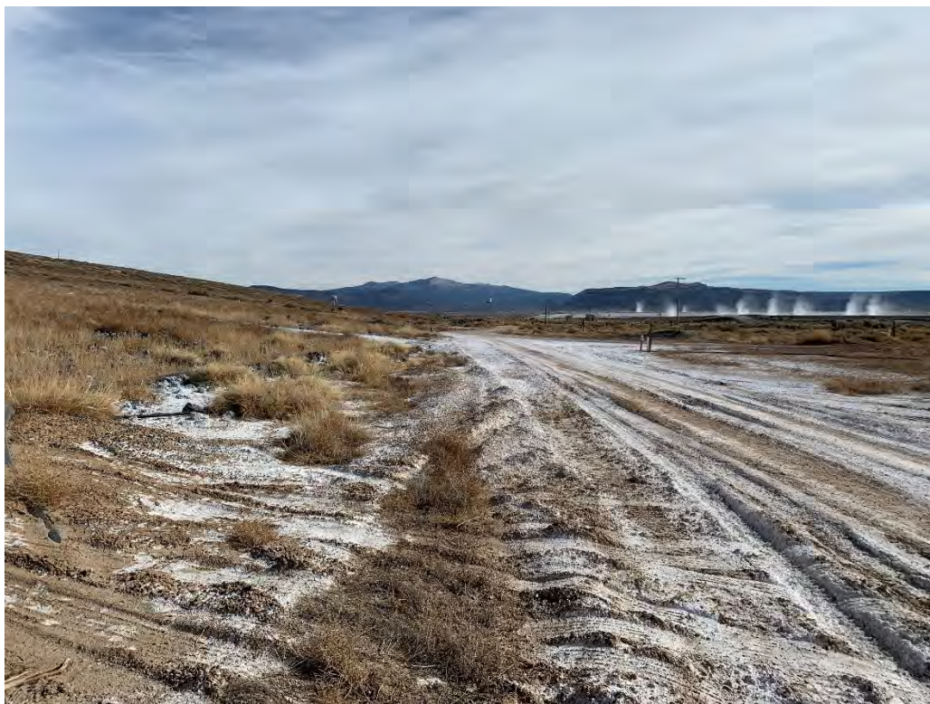
Photo 7: LTP, precipitate buildup on southwest toe and road between LTP and RO plant
