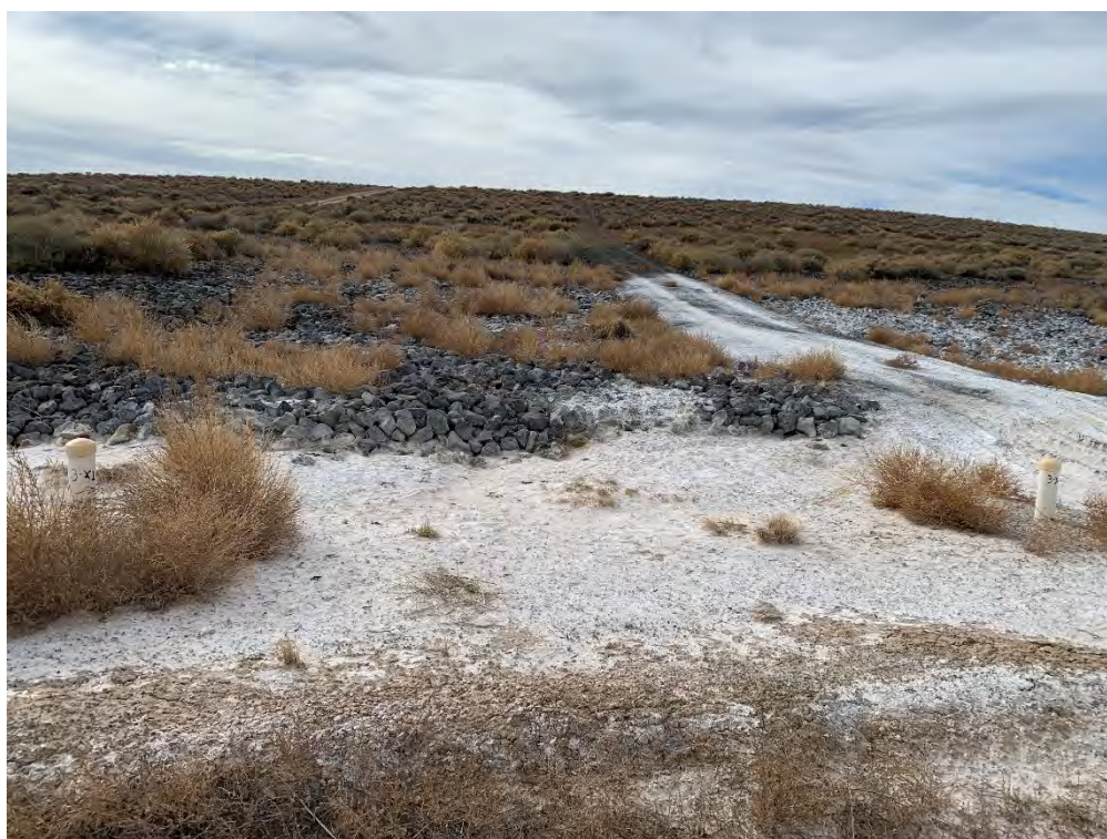
Photo 2: LTP, precipitate build up along downstream toe of north side slope
