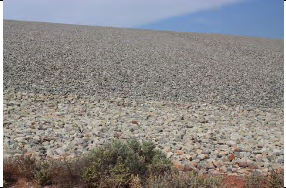
Photo 2 Northeast slope depressions in foreground
