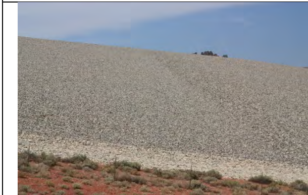
Photo 5 Change in rip rap size diagonally across northeast slope
