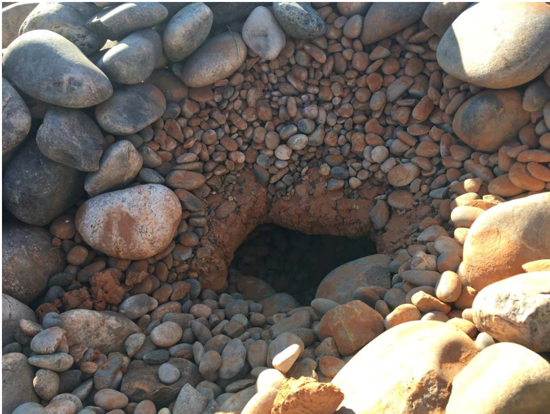
Void near toe of northeast side slope
