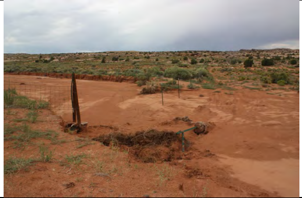
Photo 4. Main drainage sheet flow damage to northern fence crossing
