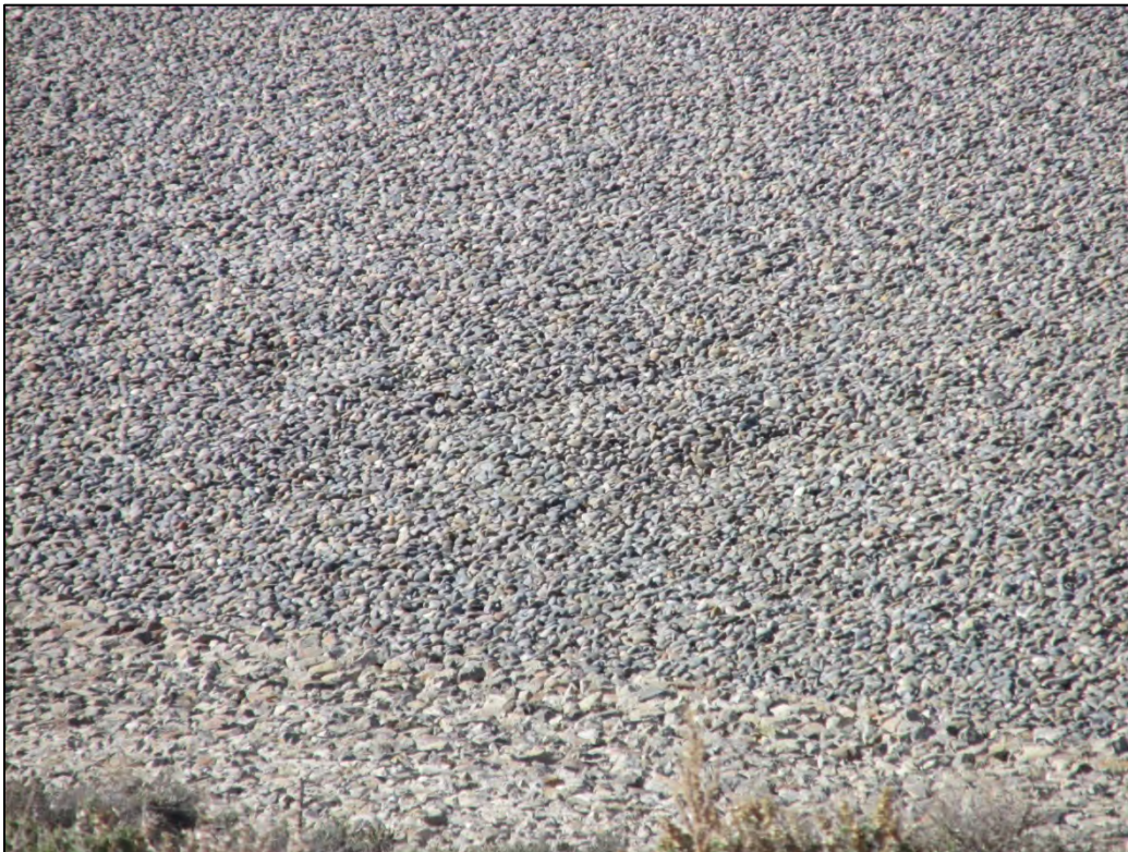
PL-10. Depressions on Northeast Side Slope Near the Toe of Disposal Cell
