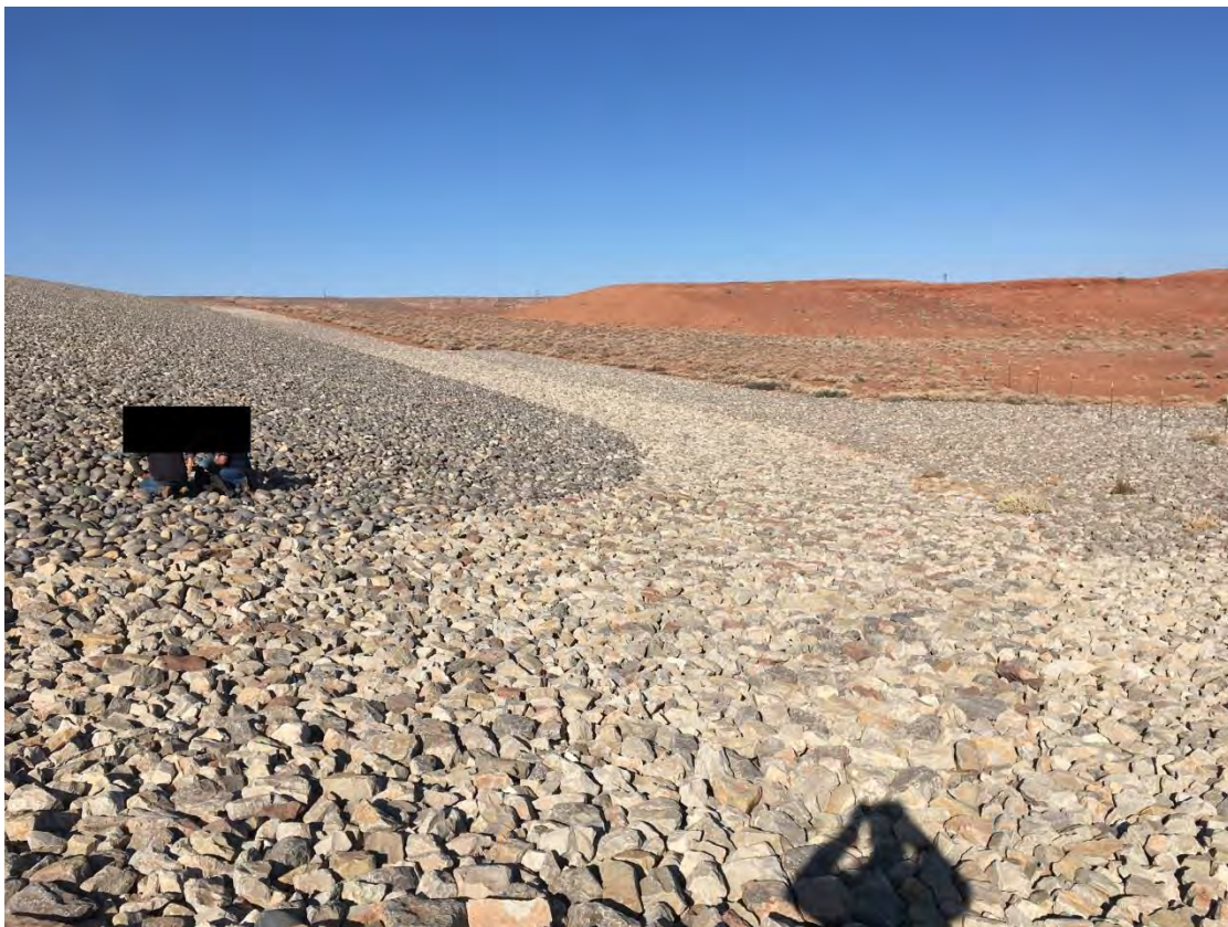
Location of void relative to toe of northeast side slope
