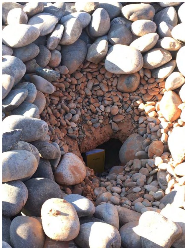
Void near toe of northeast side slope
