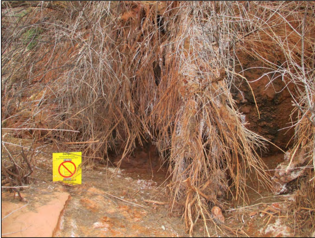
PL-21. Seep 0248 (Dripping) with Partially Buried Warning Sign
