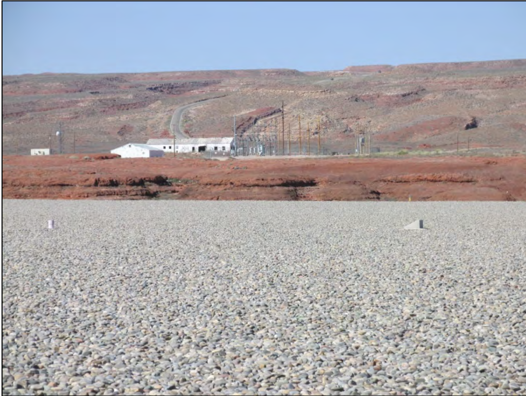
PL-7. View West Across Disposal Cell Top Slope With Site Marker SMK-2
