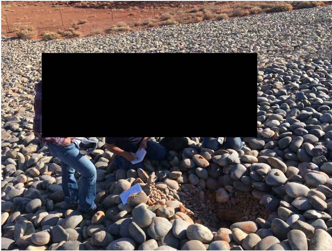
Relative location of void beneath small area of hand removed rip rap and bedding material
