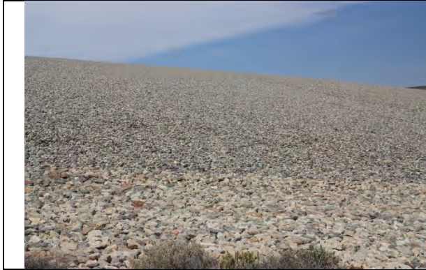
Photo 1 Northeast slope depressions in foreground
