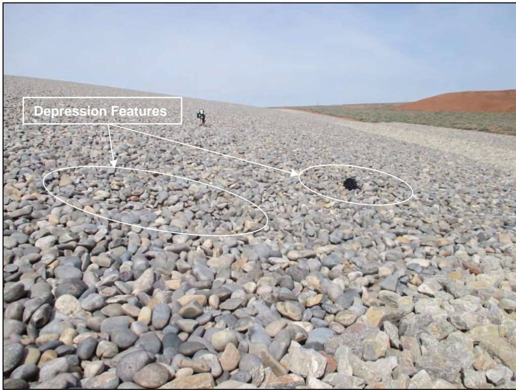
PL-9. Depression Features near Toe of Northeast Side Slope (Black Backpack for Scale)
