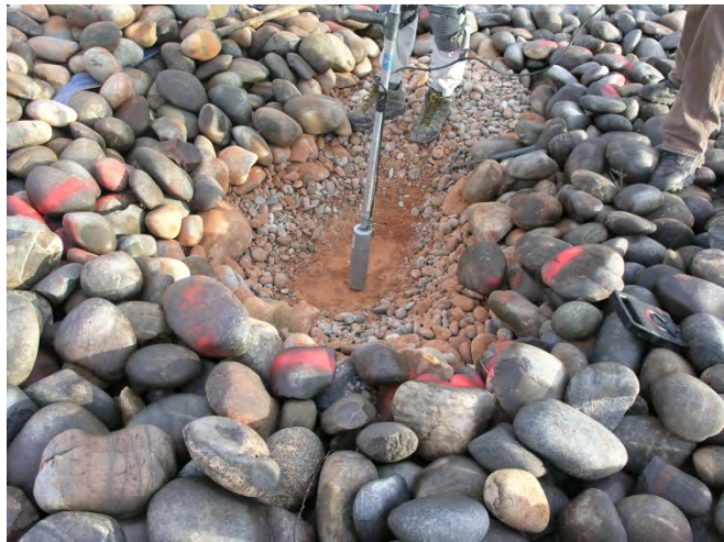
TP8 – Top of Radon Barrier
