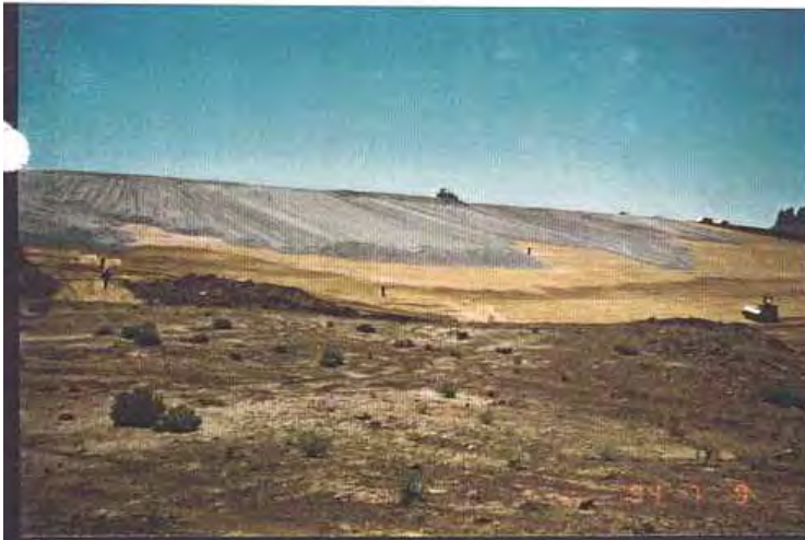
Cell, overview of northeast 5:1 slope radius area: Bedding material application activities over approved radon barrier material surface.
