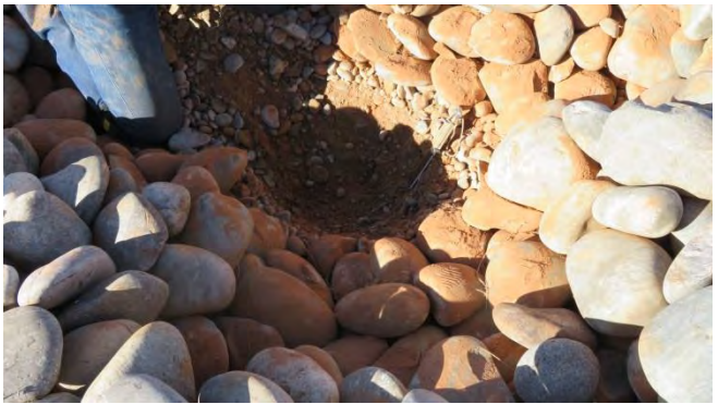
TP11 – Top of Radon Barrier
