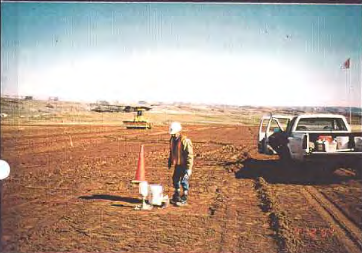
Cell, west 2% slope area: QC testing — Sandcone density test on second of three lifts of radon barrier material.
