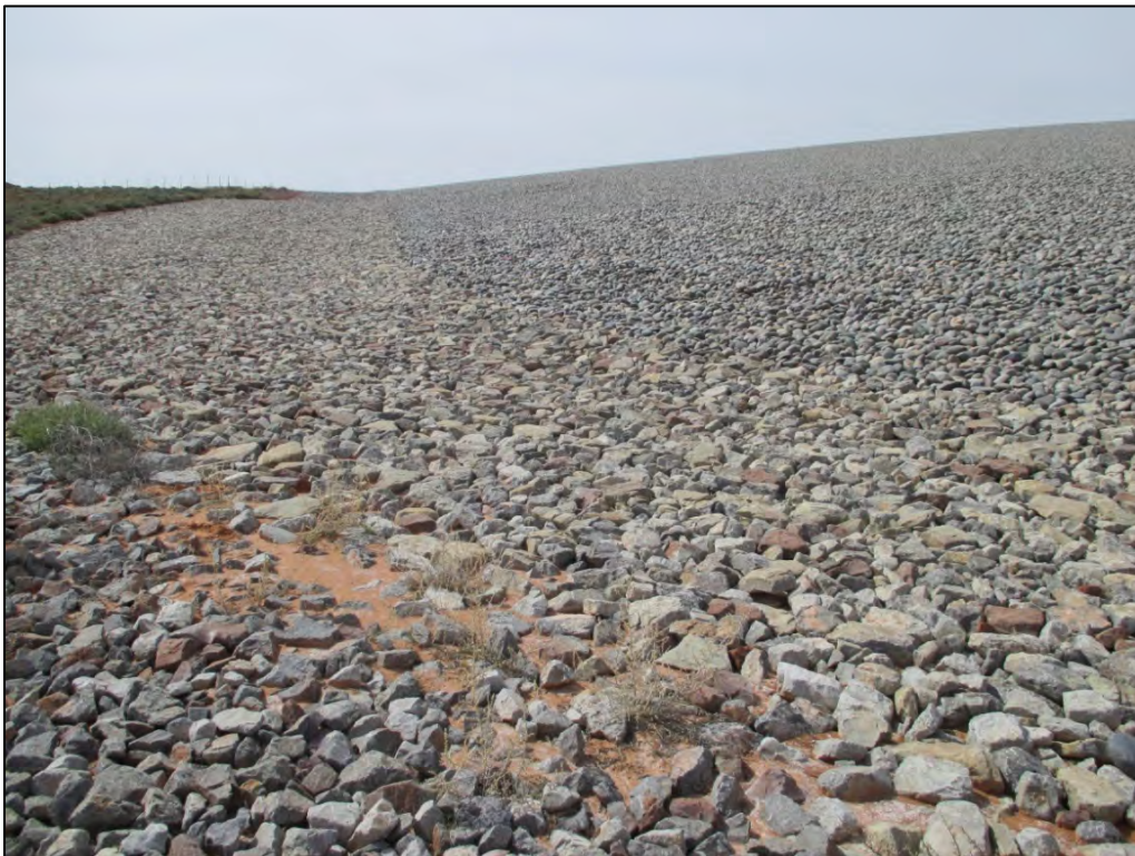
PL-14. Sediment Accumulation Along Transition Zone from Apron to Northeast Toe Drain; View to the South
