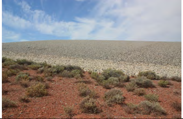
Photo 4 Change in riprap size diagonally across northeast slope
