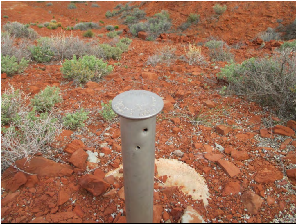
PL-7. Boundary Monument BM-5 with Bullet Damage
