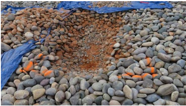
TP12 – Top of Radon Barrier
