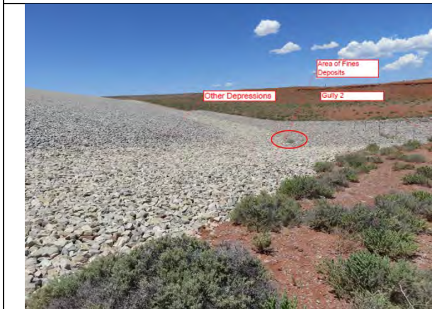
Photo 15 - Rock Drain Low Point
