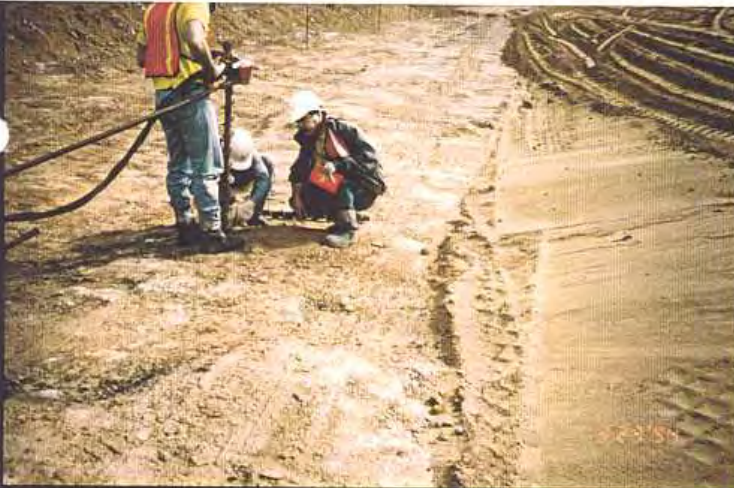
Hat Site, north side - toe of 5:1 slope: QC personnel, verification of competent in-situ rock — Drilling to refusal with auger drill.
