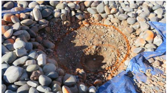
TP10 – Top of Radon Barrier
