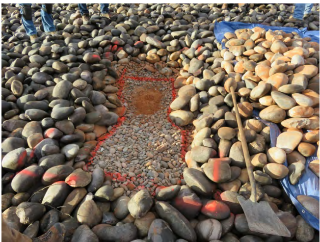
TP8 – Bedding Layer and Top of Radon Barrier
