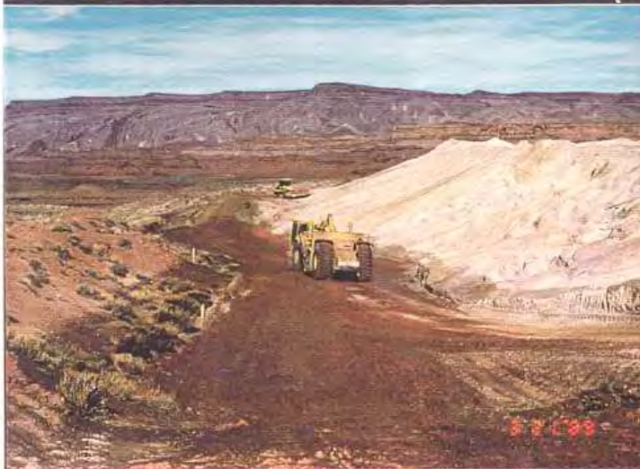
Cell, 5:1 slope area; Cat 631 scraper, delivering and spreading contaminated windblown material.
