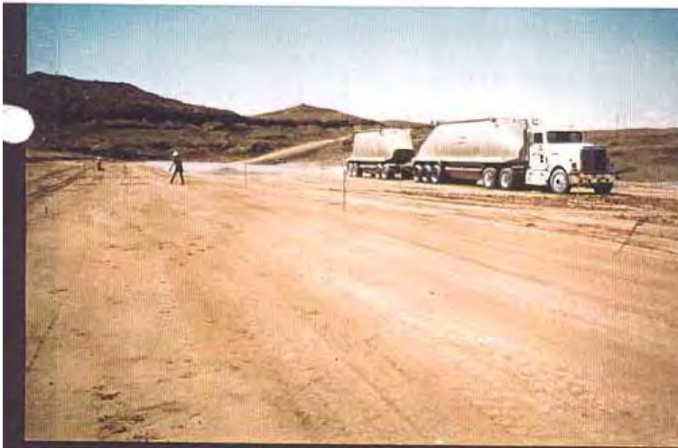
Cell, overview of 2% slope area: Semi-trailer-pup belly-dump, delivering bedding material over approved radon barrier material surface.
