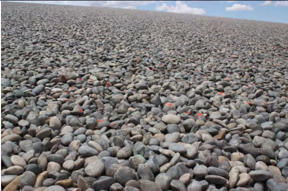
Photo 24 Red outlines of depressions near the toe of northeast slope and Gully #2
