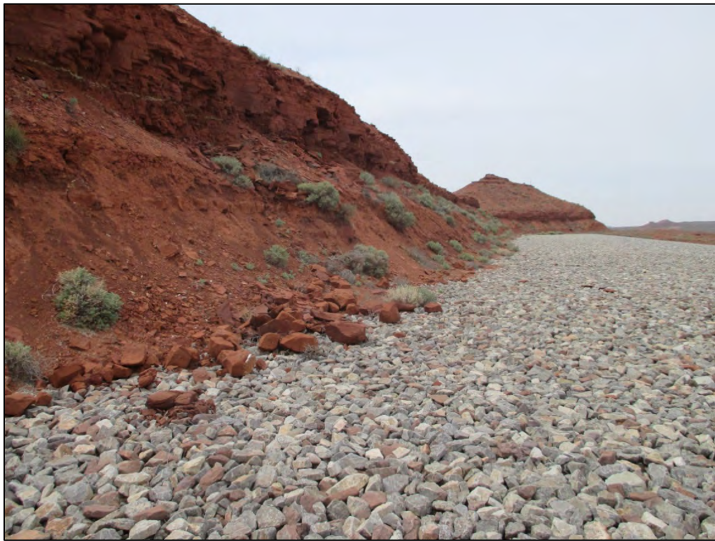
PL-10. Sloughed Rock on Riprap Apron near South Slope of Disposal Cell
