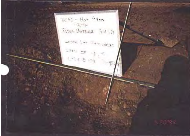
Cell: QC verification, third (final) lift of radon barrier material — Loose lift thickness check.
