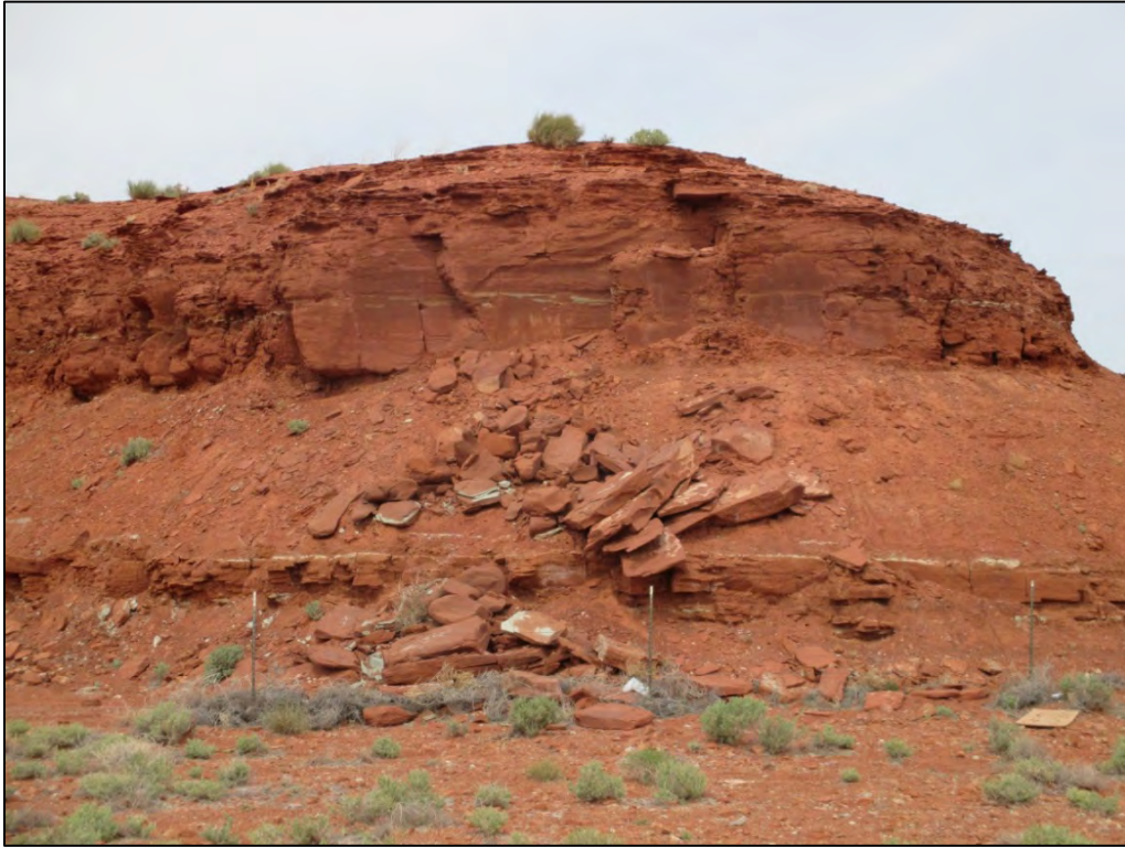
PL-15. Sloughed Rock Approaching Fence
