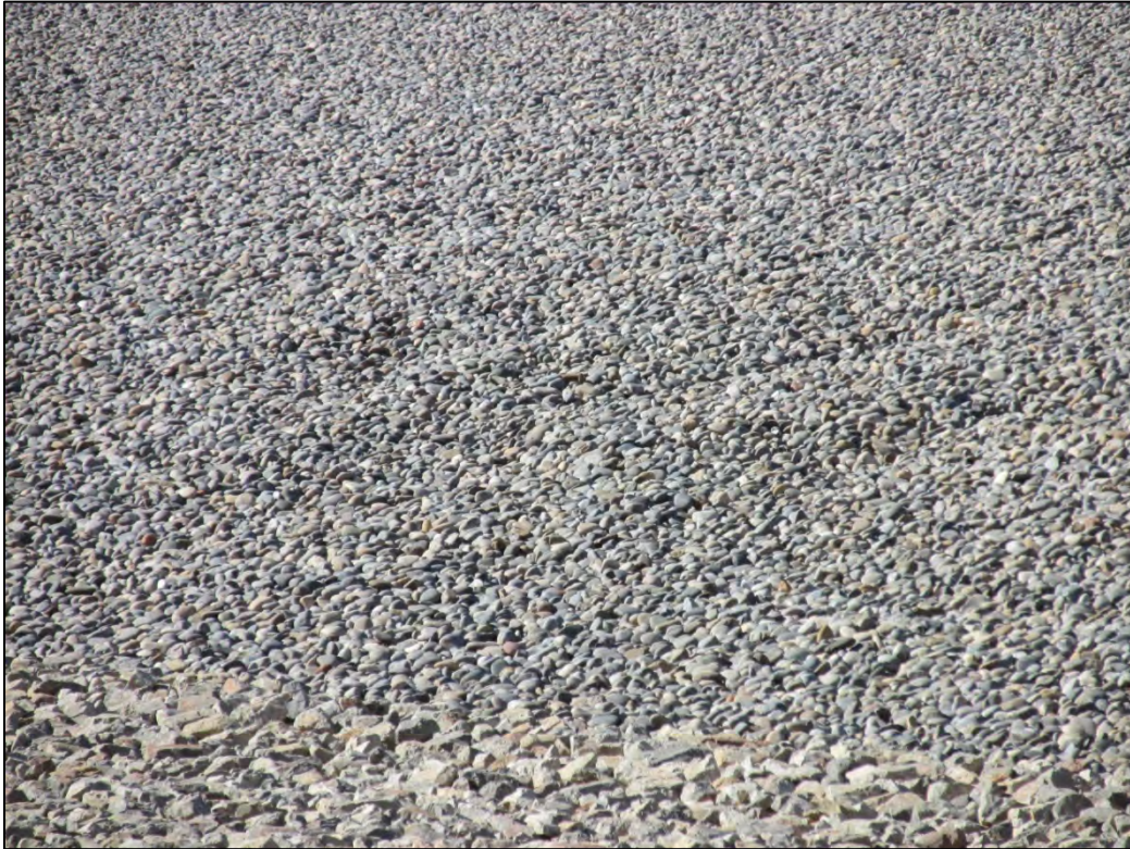
PL-11. Depressions on Northeast Side Slope Near the Toe of Disposal Cell
