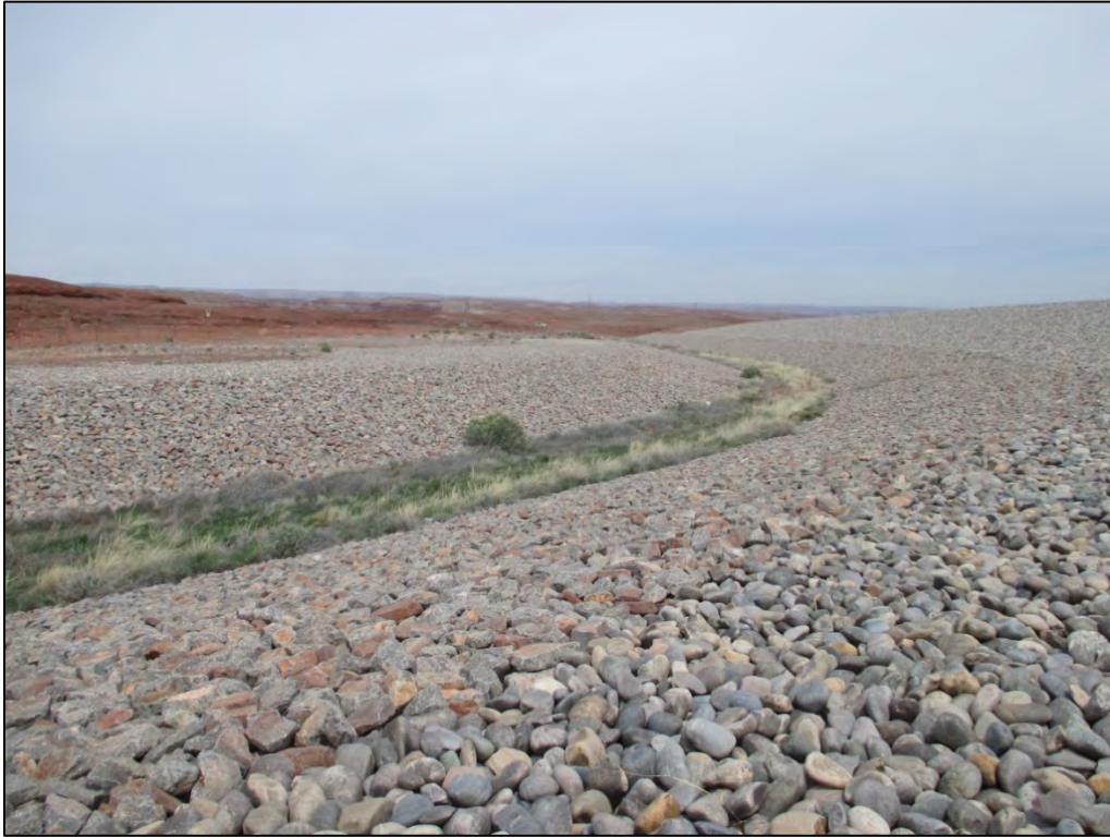
PL-13. West Diversion Channel with Vegetation Along Low Points of Drainage
