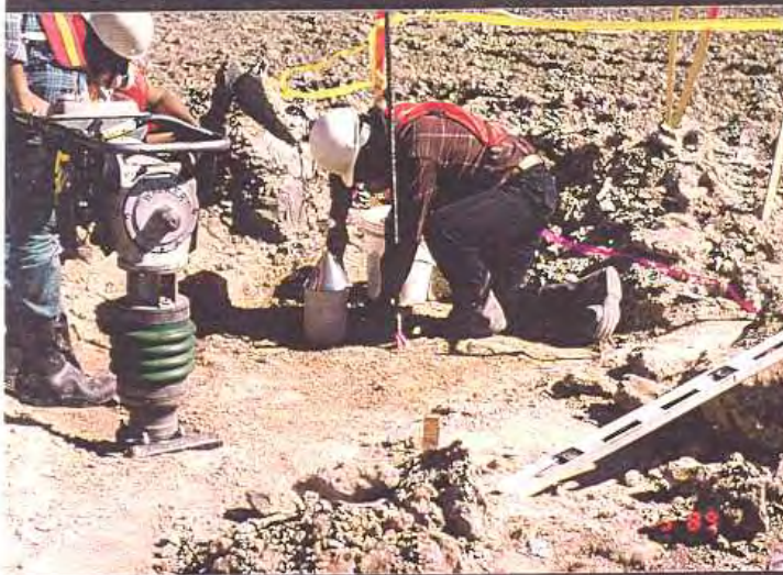
Cell, Displacement monument: After compaction of tailings placed over foundation base — QC monitoring, sandcone density test.
