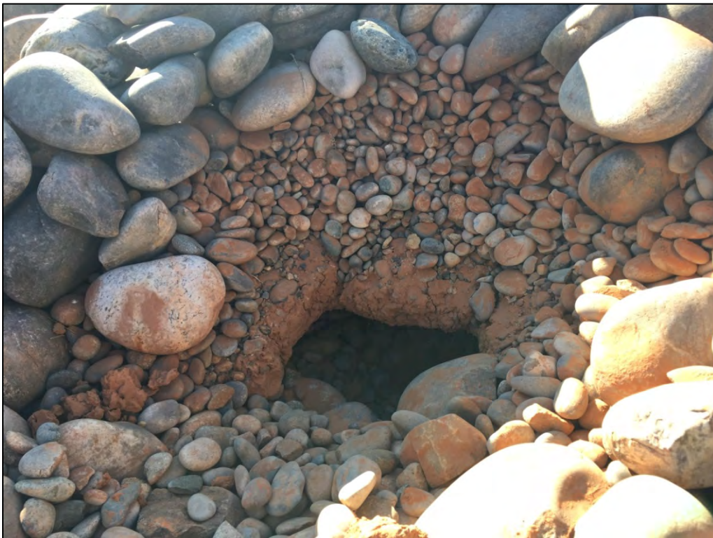
PL-12. Void Along Bedding Layer and Radon Barrier Interface (Observed During December 14, 2017 Site Visit)
