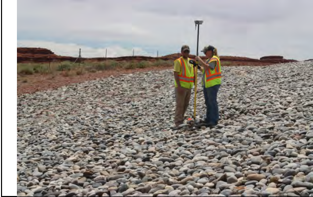
Photo 19. Surveyors gathering data on existing depressions on the northeast side slope of the Mexican Hat Disposal Cell
