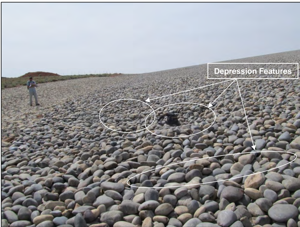
PL-8. Depression Features near Toe of Northeast Side Slope (Black Backpack for Scale)
