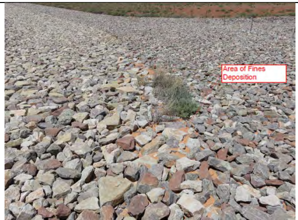
Photo 16 – Rock Drain Low Point
