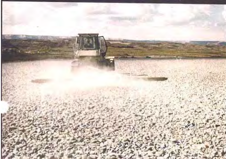
Cell, 2% slope area: Dozer / weighted pipe, final grading of type A erosion protection material surface.
