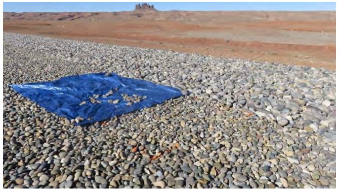
TP9 – Top Slope Riprap
