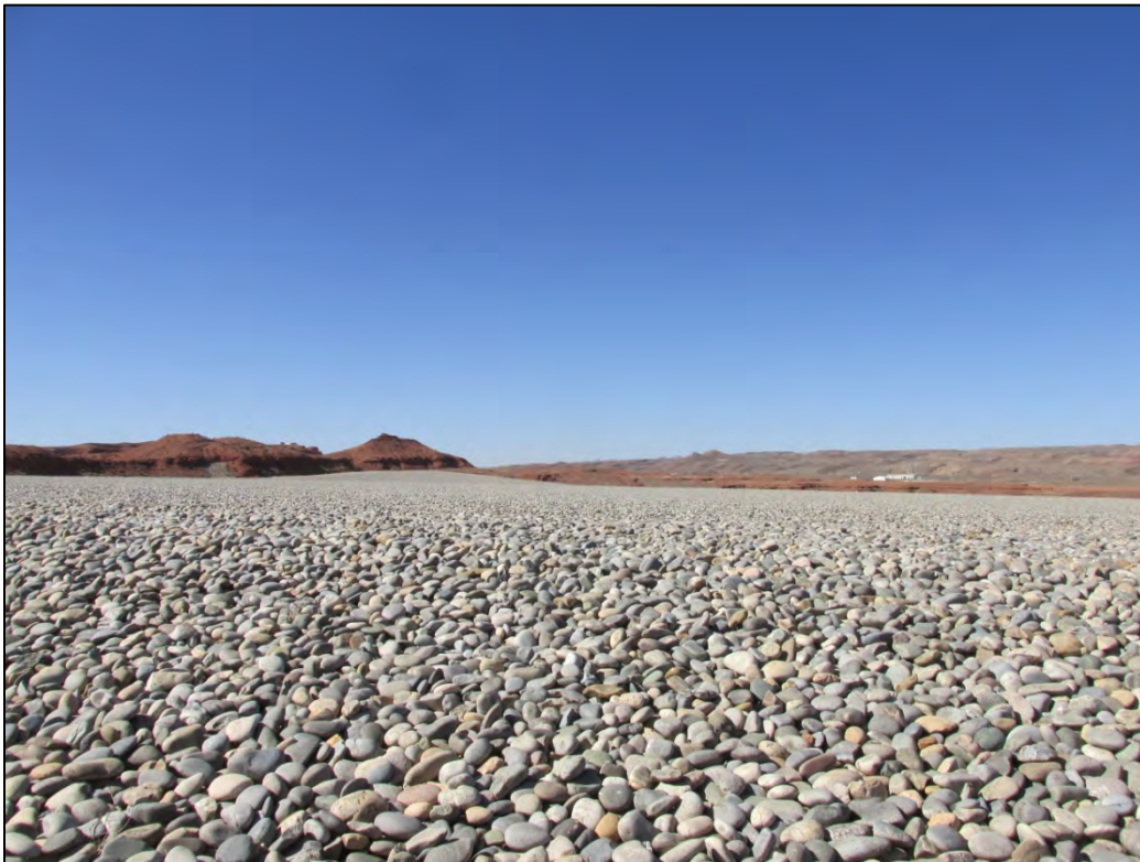
PL-6. View Northwest Across Disposal Cell Top Slope
