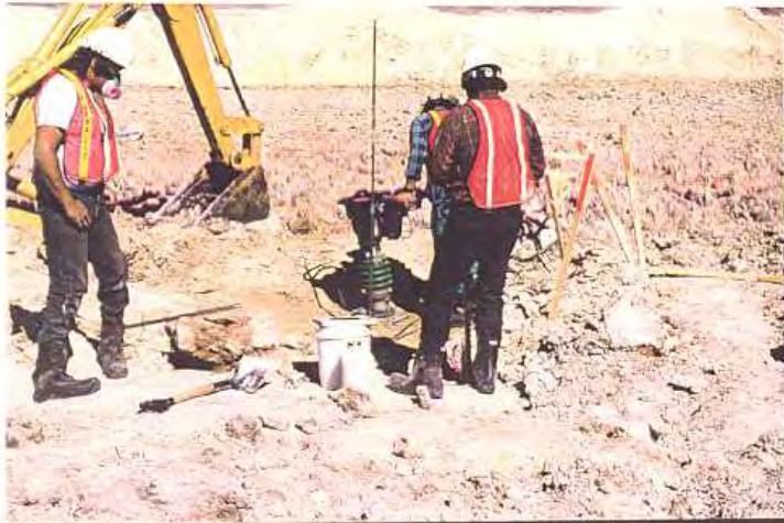
Cell, Displacement monument: Contaminated tailings placed over foundation base — Compaction effort.
