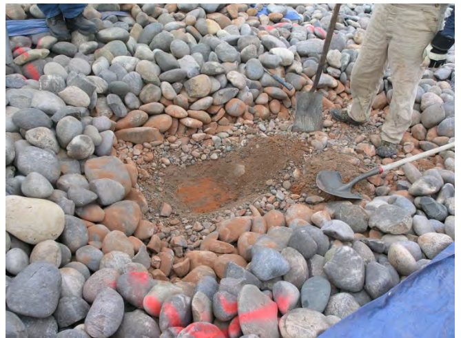
TP4 – Top of Radon Barrier
