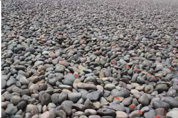
Photo 21 Red outlines of depressions near the toe of northeast slope and Gully #2
