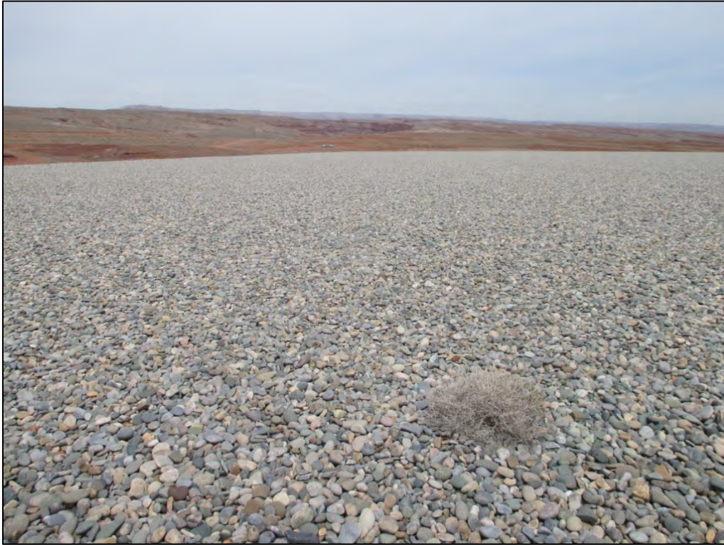
PL-11. Fourwing Saltbush on Top Slope of Disposal Cell (Removed)
