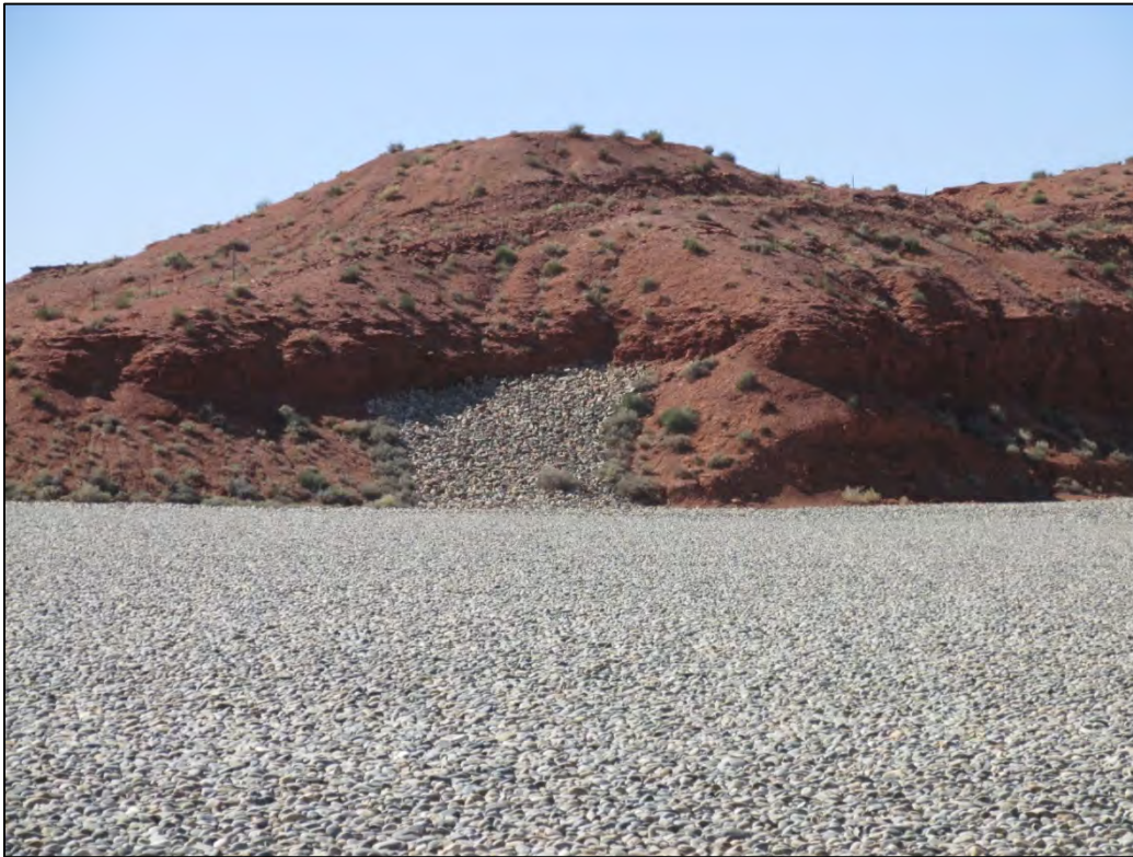
PL-9. Sloughed Rock Area Along South Edge of Disposal Cell
