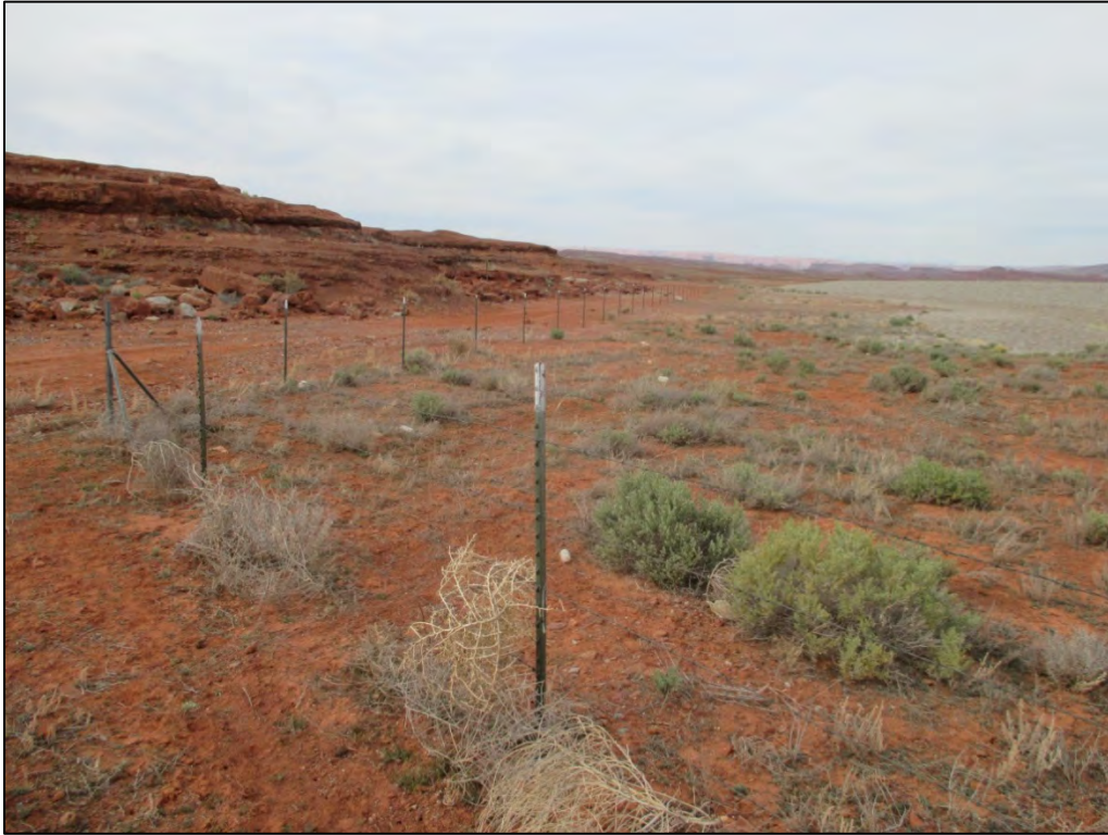
PL-3. Fence Enclosing Southwest Portion of Disposal Cell
