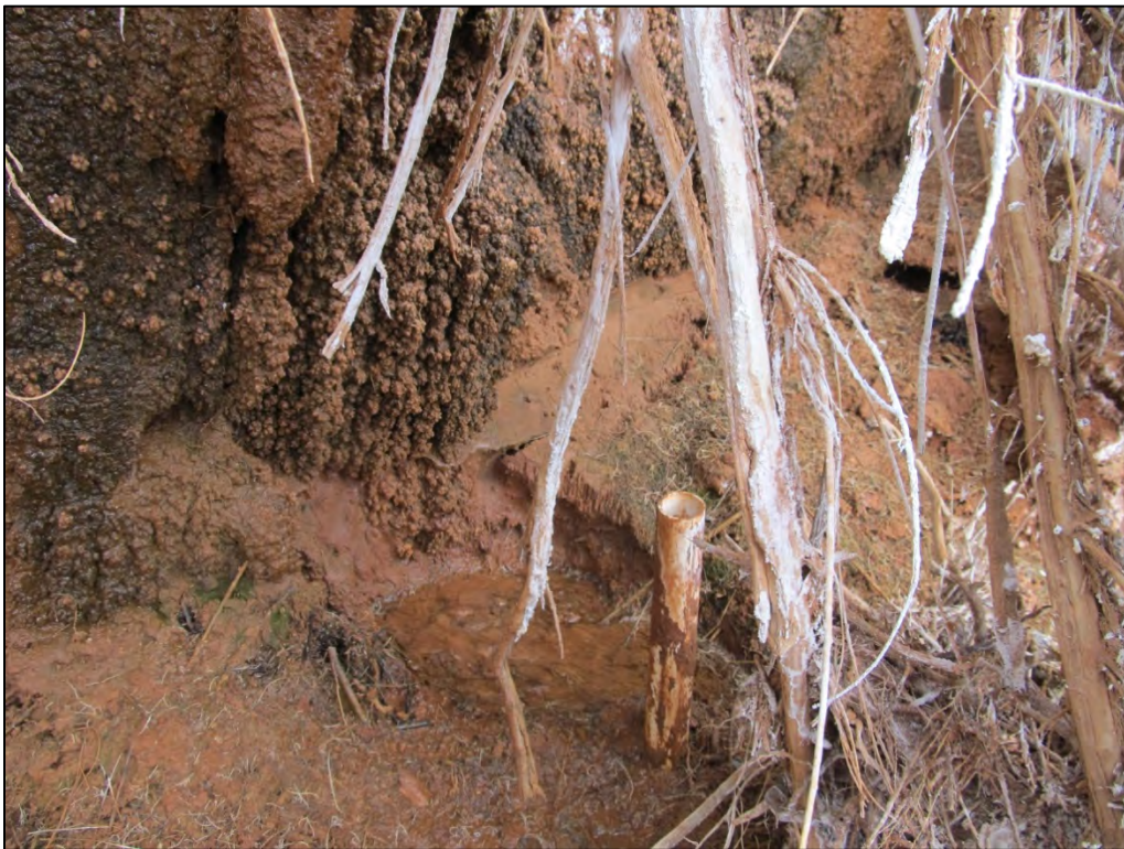
PL-22. Seep 0248 (Dripping) with Pooled Water at Base of Cliffside
