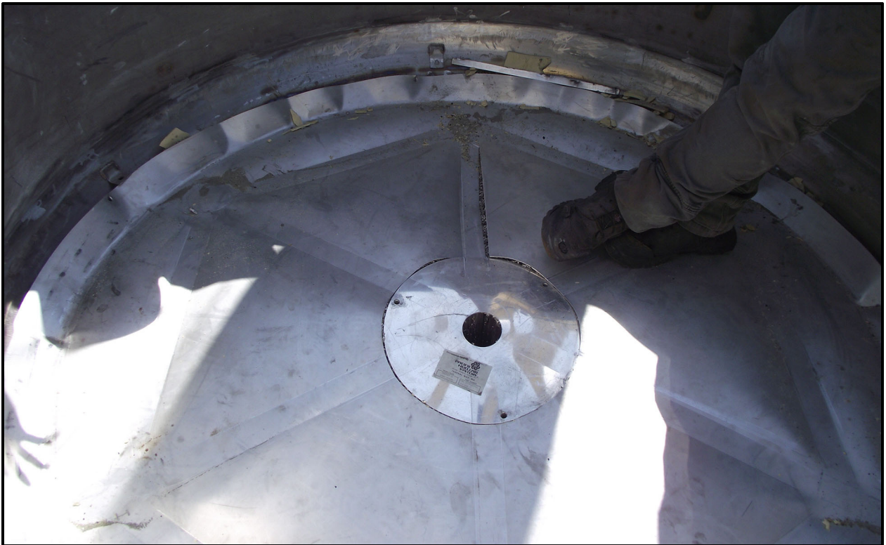
Figure 6-31 – SC-30G3 Deformed Lower Spacer
