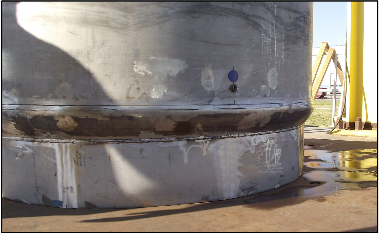
Figure 6-5 – SC-55G1 End Drop Hoop Damage to the ICV Shell
