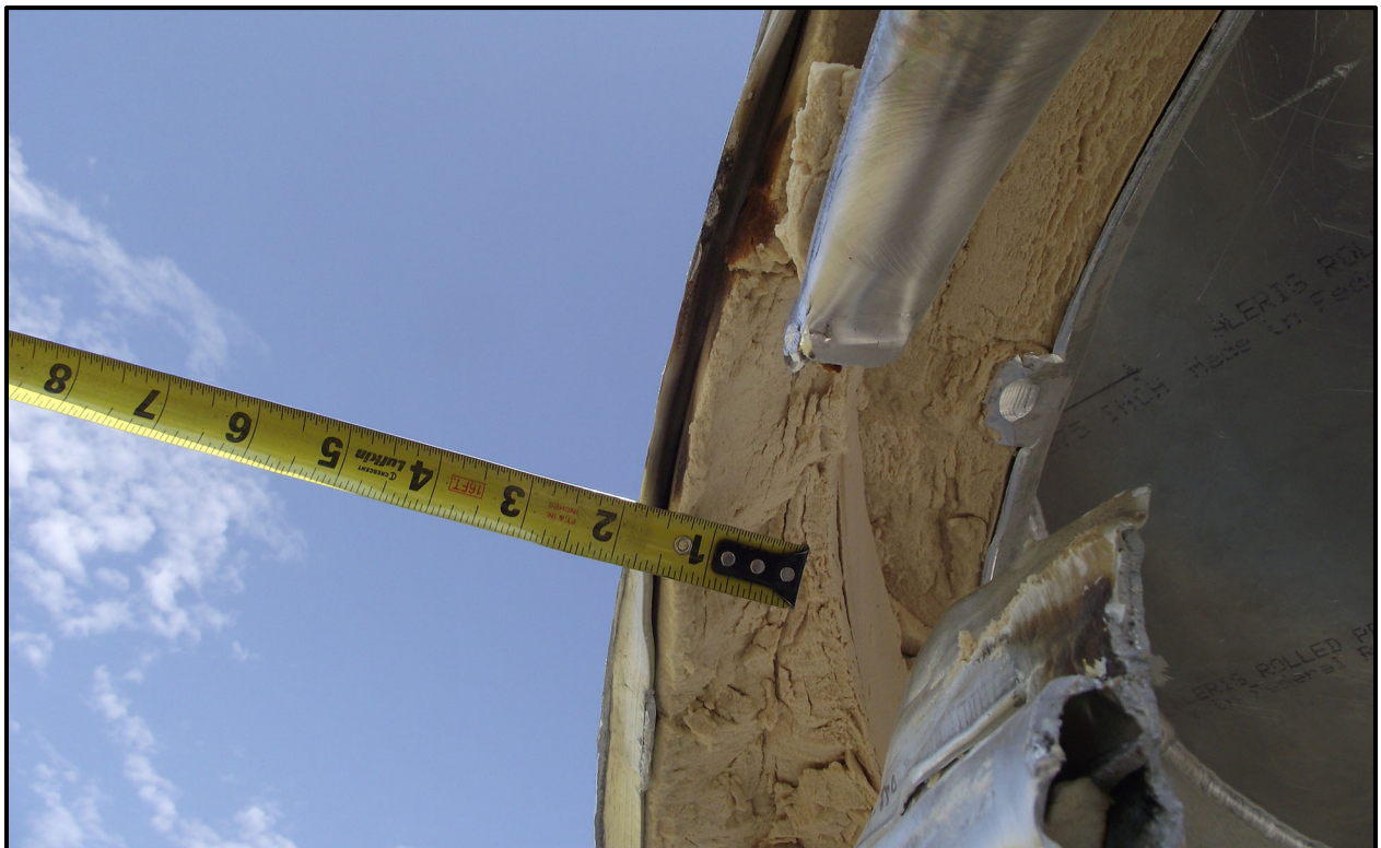
Figure 6-16 – SC-55G1 Radial Dunnage Upper-End Residual Thickness
