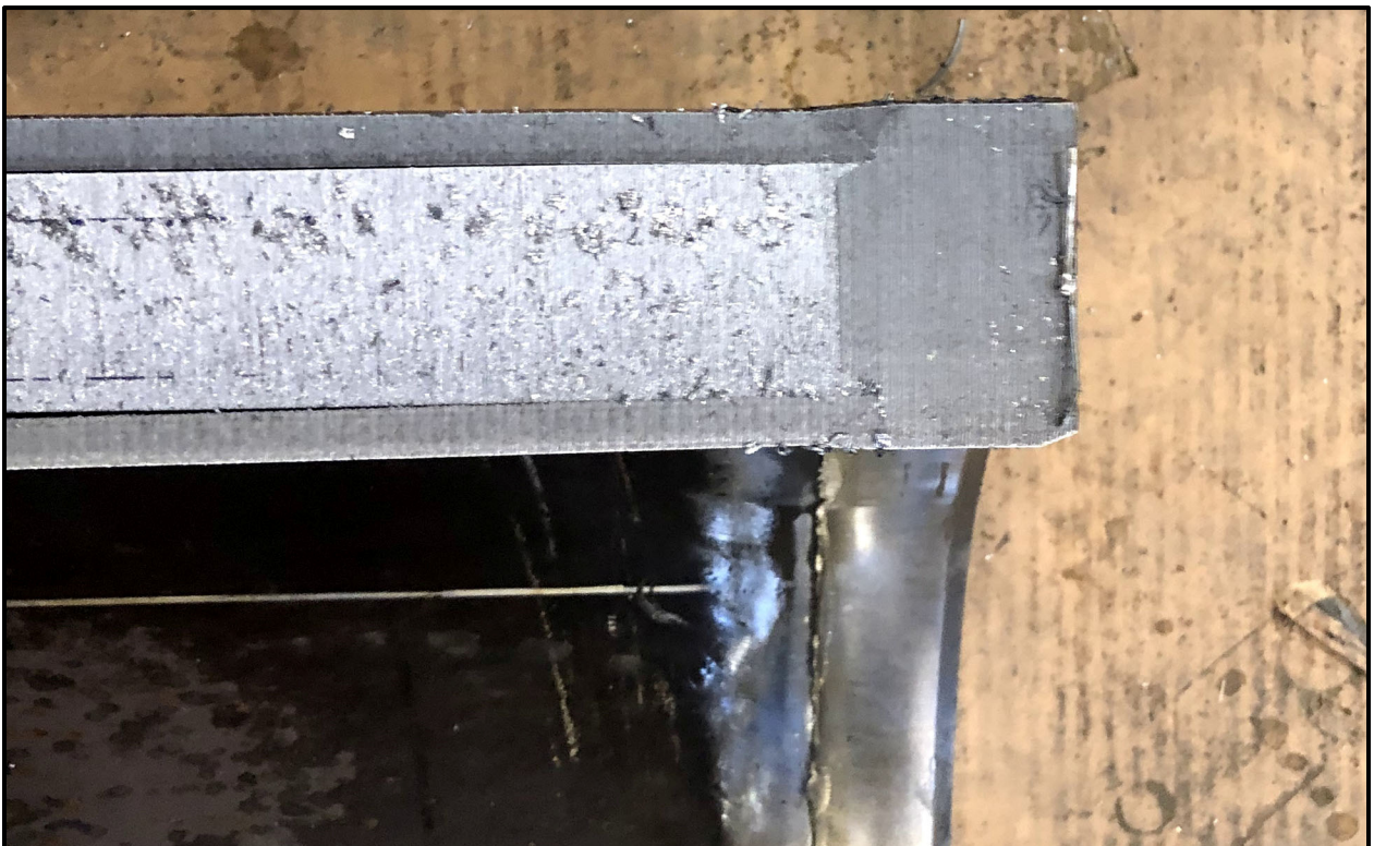
Figure 7-17 – SC-30G2 18TU-02 Destructive Disassembly Cut AT/AU at Upper Flange
