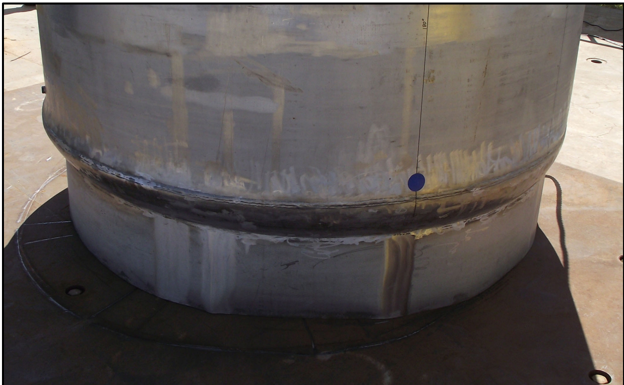
Figure 6-25 – SC-30G3 End Drop Hoop Damage to the ICV Shell
