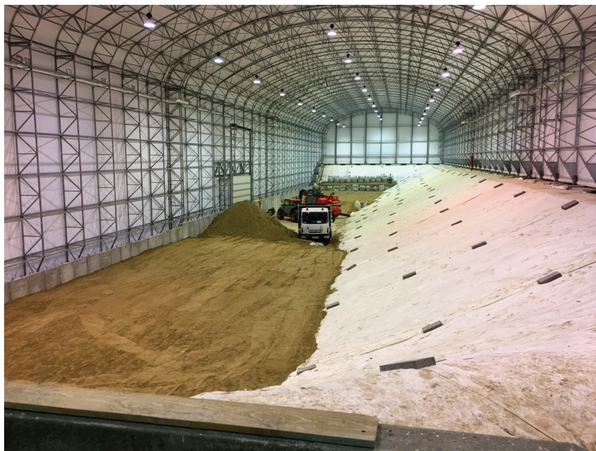
FIGURE 2-6 An operational disposal site for very low-level waste (VLLW). This facility is one cell (approximately 150 meters in length, 40 meters in width with a capacity of 30,000 cubic meters). Note the small gray cubes at back of facility; each is one cubic meter of VLLW.
