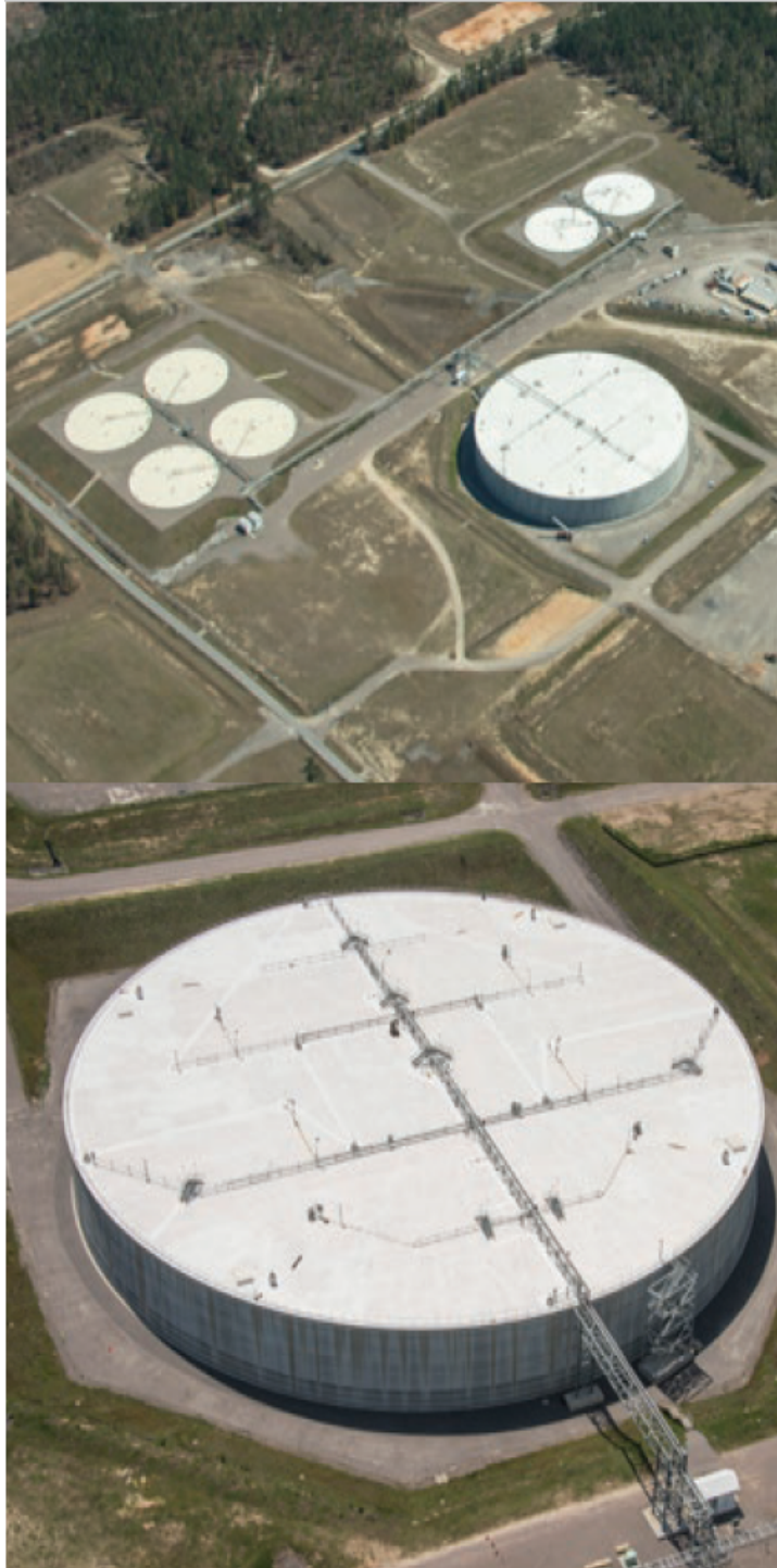
Figure 3-11. Saltstone disposal units: Closeup of the 121-million-L [32-million-gal] unit in the bottom image and all the units, including the smaller 11.4-million-L [3-million-gal] units in the top image (SRR, 2017)
