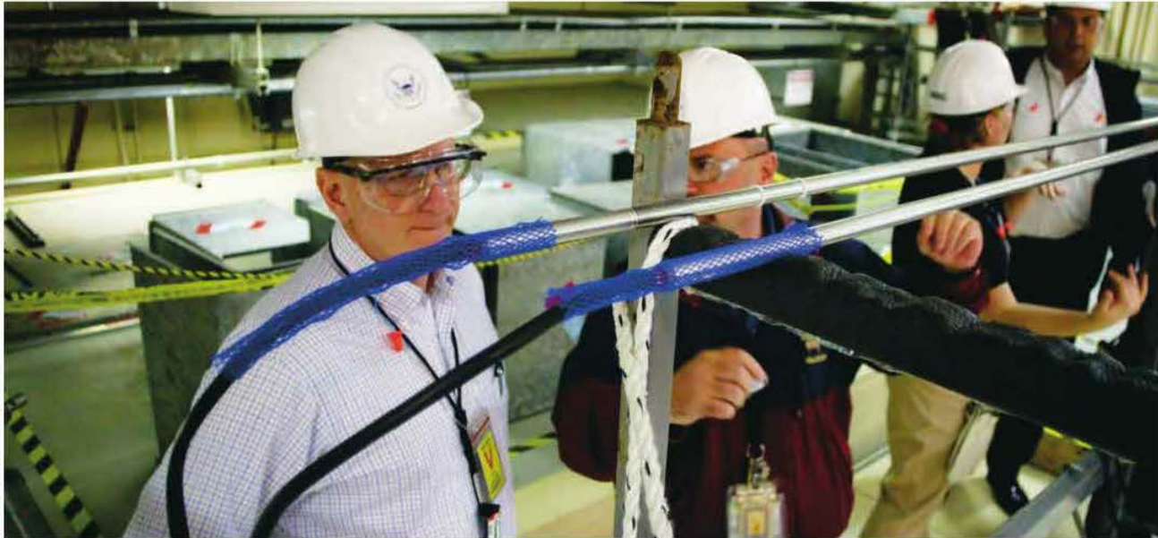
NRC Commissioner William C. Ostendorff (left) speaks with NRC Senior Resident Inspector John Kirkland about repairs needed at Fort Calhoun while touring the plant during its 30-month outage.
