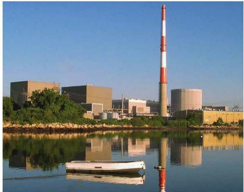
The Millstone Power Station in Waterford, CT, which experienced two self-inflicted near misses in 2014 when recent maintenance and modifications introduced problems that reduced safety margins.
