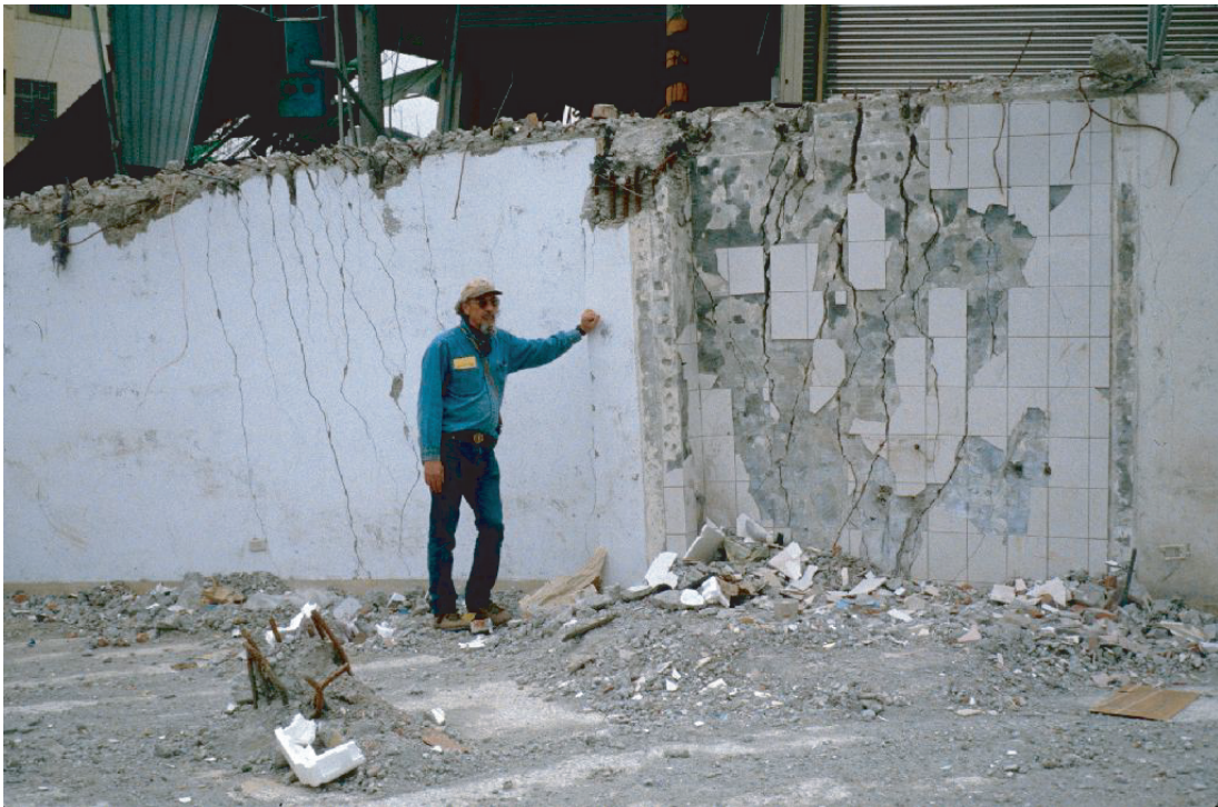
B) Shears and fractures in wall over the fault bend fold shown above.
