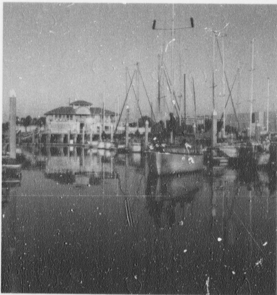
The Harborage at Bayboro, a Development Group project, features a floating concrete dock system and includes 235 private slips, 2,500 feet of dock space for visitors and a two-story dockmaster's office.
