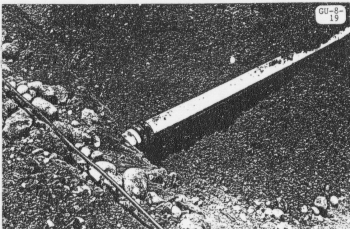
Sewer Service Line Repairs.
