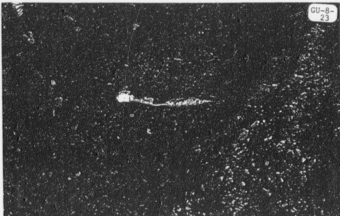
Broken Sewer Service Line to Wendell's Print Shop STA 1+50.
