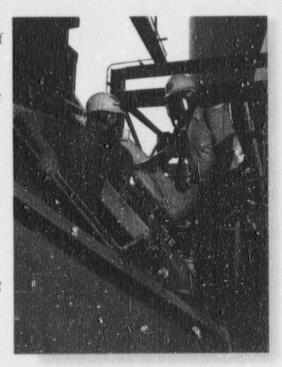
Robert Vail emerges from inspection of the SO, scrubber inodule at Gross Generating Station, assisted by fellow technician Robert Mathis, Rigid maintenance and operation of the environmental control equipment at the generating stations helps assure emissions compliance and increased operating efficiency.
