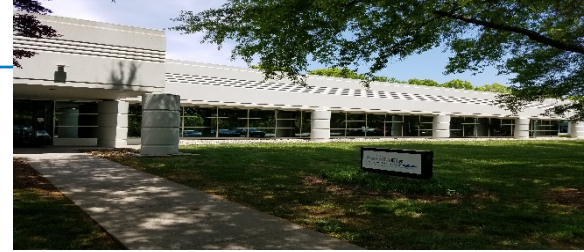
Perma-Fix Business Center Knoxville, TN
