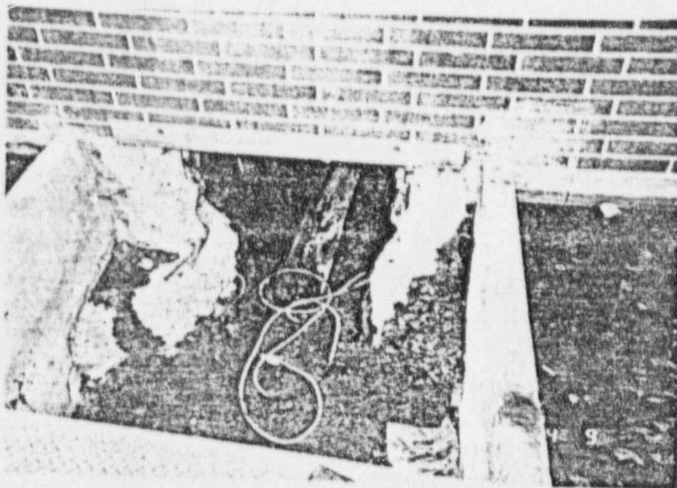
Crawl Space Access Pit Looking South
