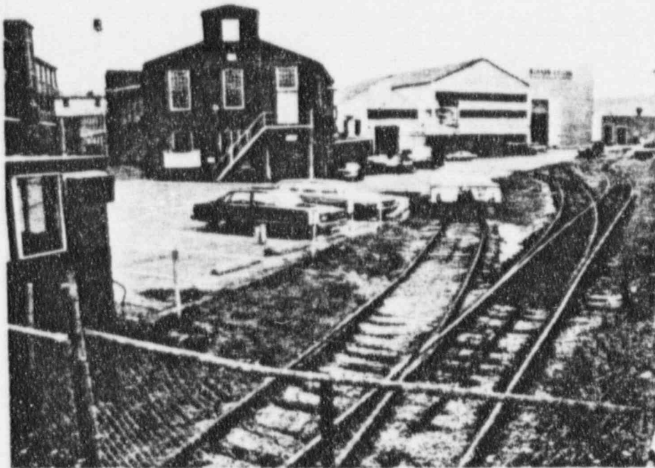
Area "A" Looking Northeast
