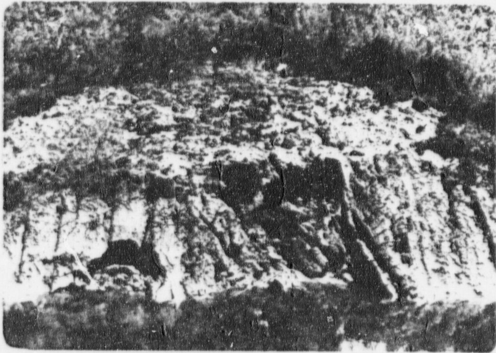
PHOTO 27 - VIEW OF FINGER DRAIN AND RESULTING EROSION AND SLOUGHING.
