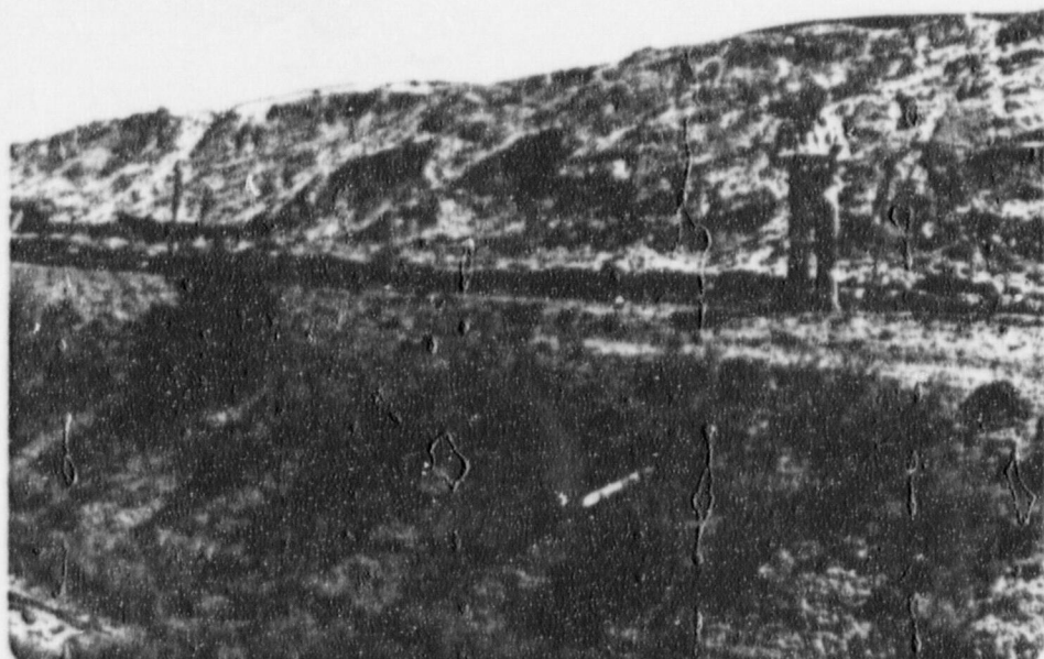
PHOTO 24 - VIEW OF SLOUCHING AND EROSION ON DOWNSTREAM SLOPE OF STAGE 1 TAILINGS DIKE.
