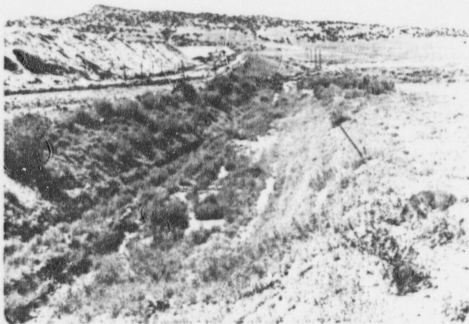
PHOTO 4 - CLOSE-UP VIEW OF DOWNSTREAM SLOPE, LOOKING FROM NORTH TO SOUTH. NOTE SEEPAGE COLLECTOR DITCH AT TOE OF STARTER DAM.
