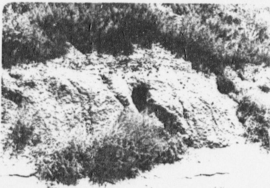
PHOTO 26 - VIEW OF FINGER DRAIN AND EROSION HOLE. NOTE POSSIBLE DISPERSIVE SOIL.
