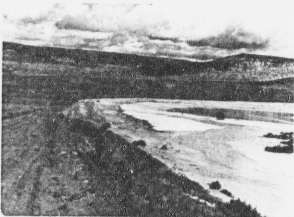
PHOTO 8 - VIEW OF CREST OF STARTER DAM (LEFT SIDE OF PHOTO) AND STAGE 1 TAILINGS DIKE, LOOKING NORTHWEST FROM SOUTH END OF STAGE 1 LIFT. NOTE BORROW AREA IMMEDIATELY IN FRONT OF STAGE 1 TAILING DIKE.
