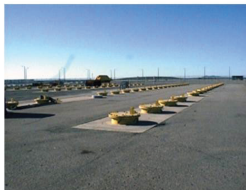
Figure 3-5. Fermi-1 blanket SNF storage at underground vaults at one facility at Idaho Nuclear Technology and Engineering Center at INEL: (a) 1 st -generation underground vaults built in 1971 and (b) 2 nd -generation underground vaults built in 1984 and 1985 (NWTRB, 2017)
