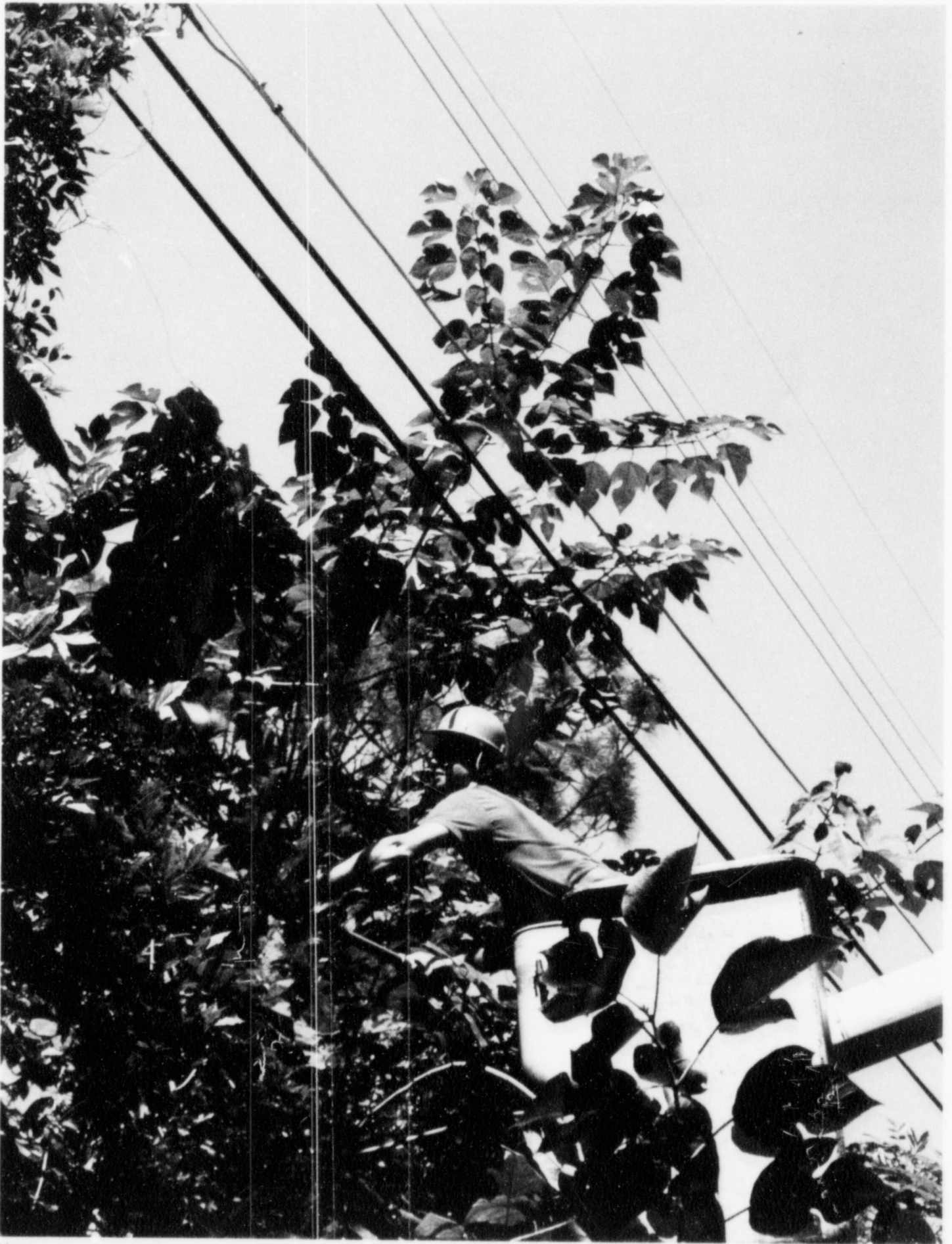
Maintenance of our 1,300 miles of 12 kilovolt overhead distribution system
