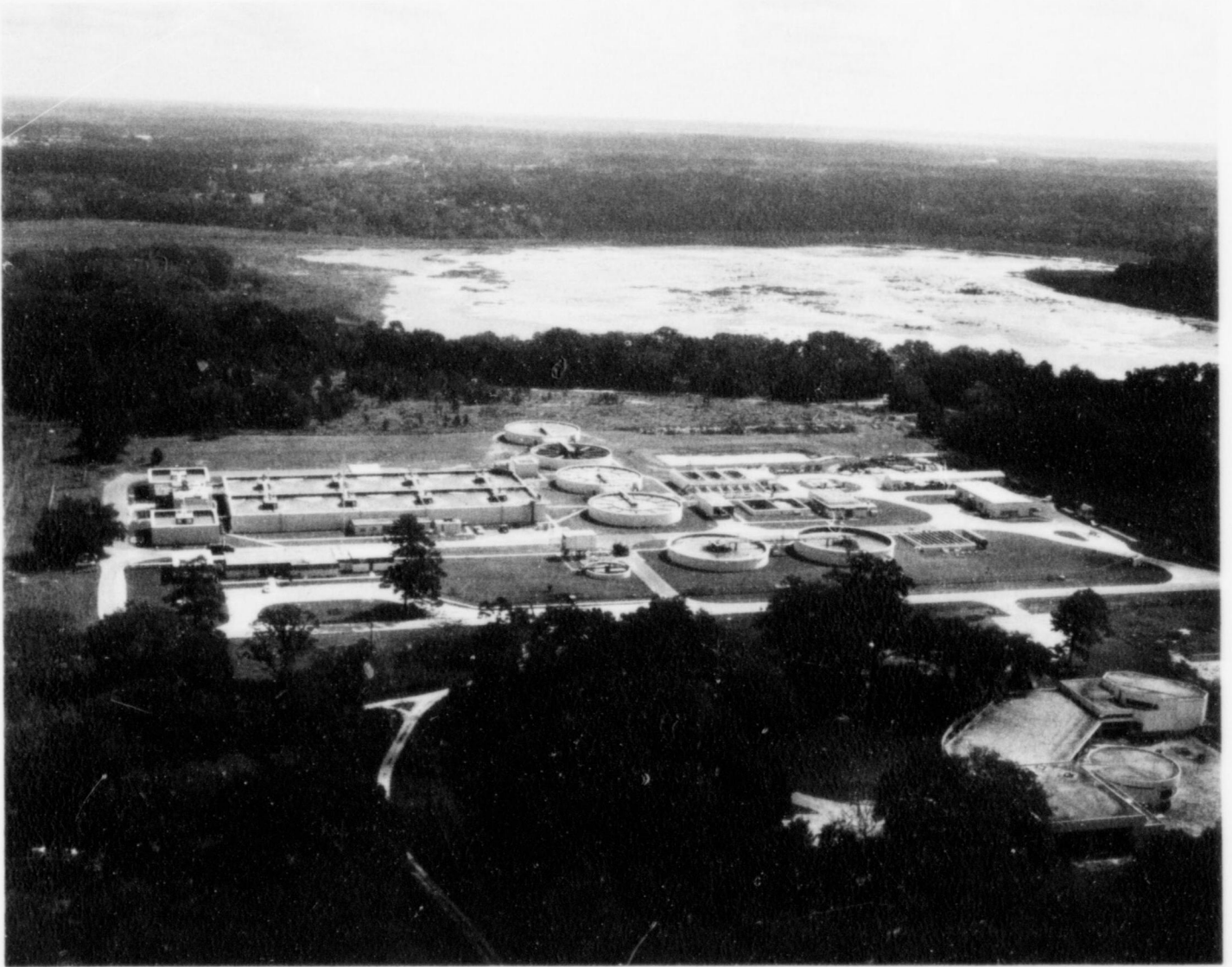
Kanapaha Wastewater Treatment Plant: ten million gallons per day treatment capacity.
