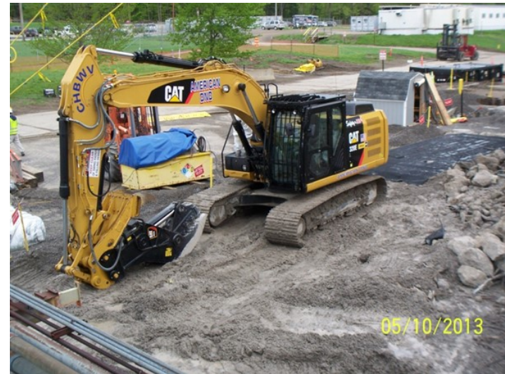
4 - 40,000 lb Class Excavator with Concrete Pulverizer
