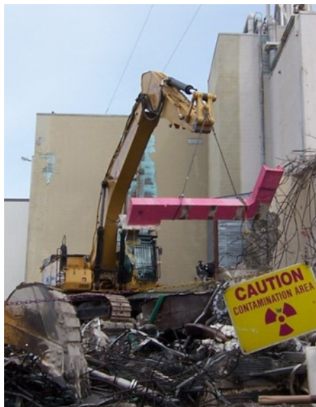
Selective Dismantling of Rad-component DURING 01-14 Demo
