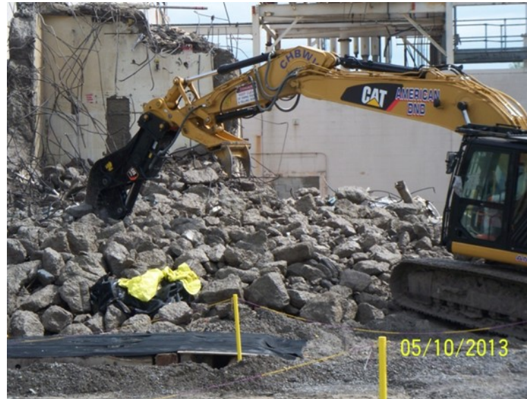
Processing and Size Reducing Concrete Rubble at 01-14
