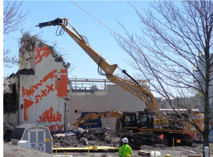
3 - 200,000 lb Class Excavator with Hydraulic Hammer (01-14 Demo)
