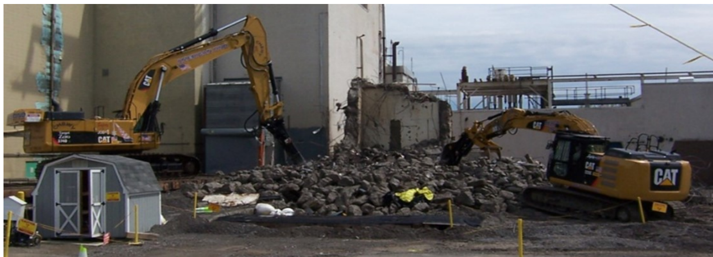
Hammer & Pulverizer Size Reducing Concrete Rubble (01-14 Rubble Pile)
