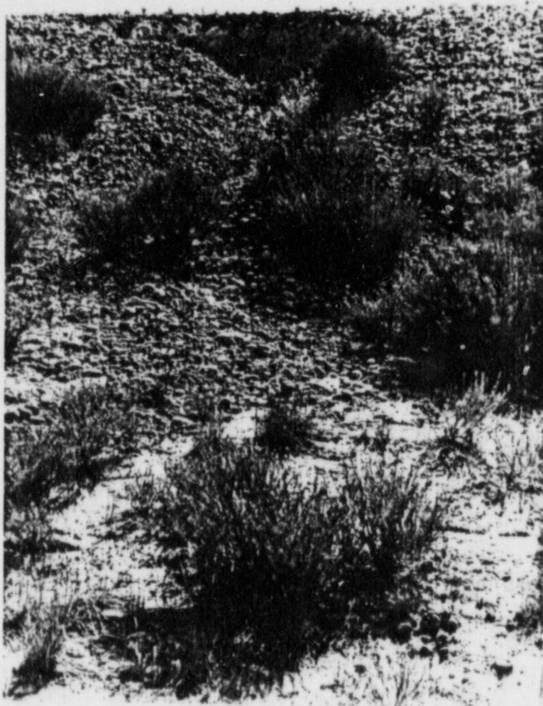
Figure 8.1 Gully breaching gravel cover along west edge of tailings pile. Headcut is about 3 feet high. Note redeposited tailings in foreground.
