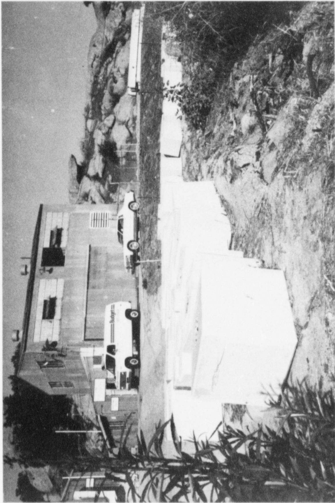
FIGURE 2: Building T-093. The high bay area of Building T-093 housed the L-85 reactor, and the low wing attached to the left served as the control room.
