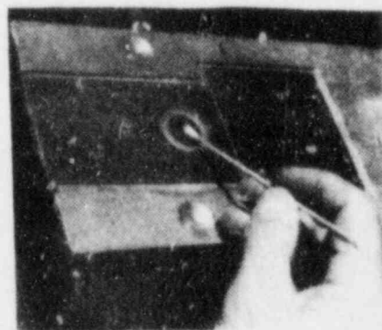
LEAK TESTING MODEL BRC MK II GAUGE AND CESIUM SOURCE OF A ANY MC SERIES GAUGE
