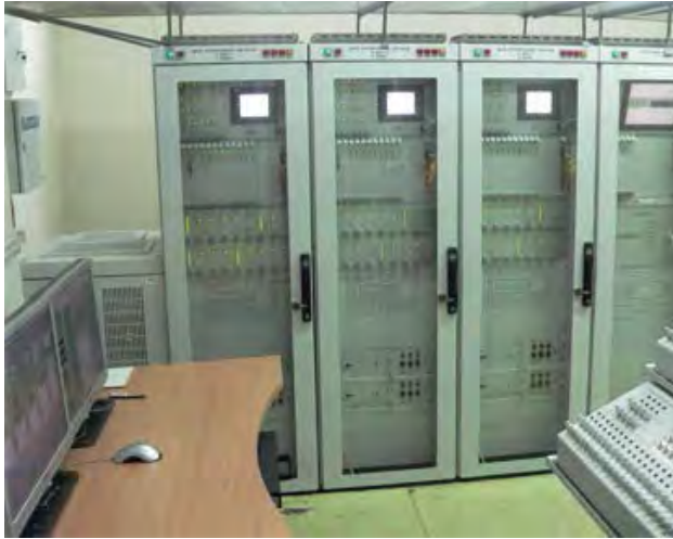
Figure 2-5: Typical RadICS Reactor Trip System Equipment
