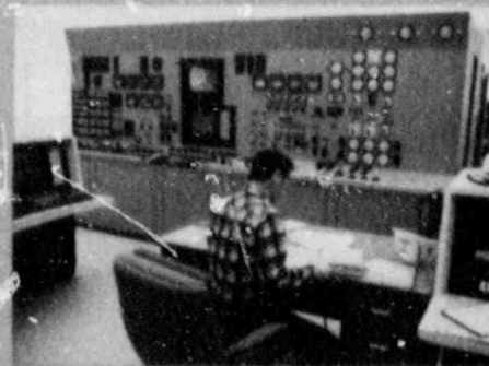
Control room at gas-fired plant
