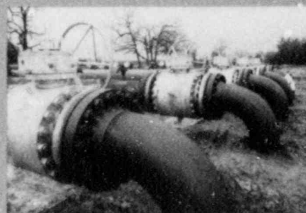
Gas pipeline addition
