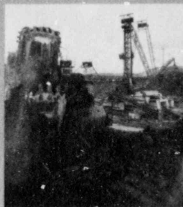
Mining lignite with the cross pit spreader
