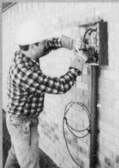
Distribution line work
