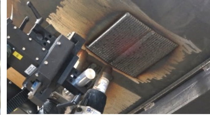
Dual GMAW for Large-Scale Heat Exchanger Overlay Repair
