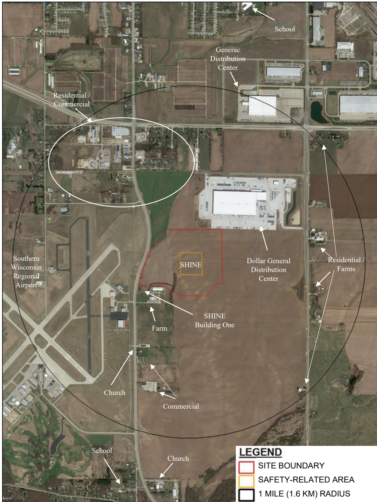
Figure 3 – SHINE Site Buildings and Surrounding Area
