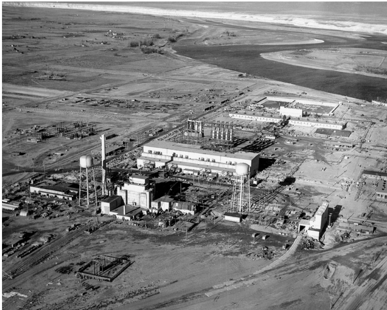
Crud was a term used early by the Hanford Engineering Works. Seen here is the site's F Reactor complex under construction. Photo courtesy of the Department of Energy
