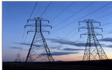
Power Transmission Equipment
