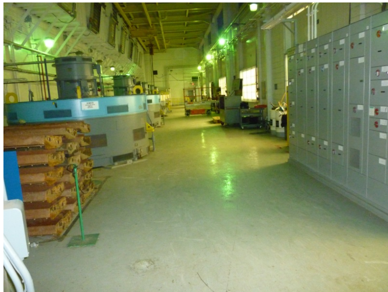
PICTURE 1 CRIB HOUSE 559 FT ELEVATION
