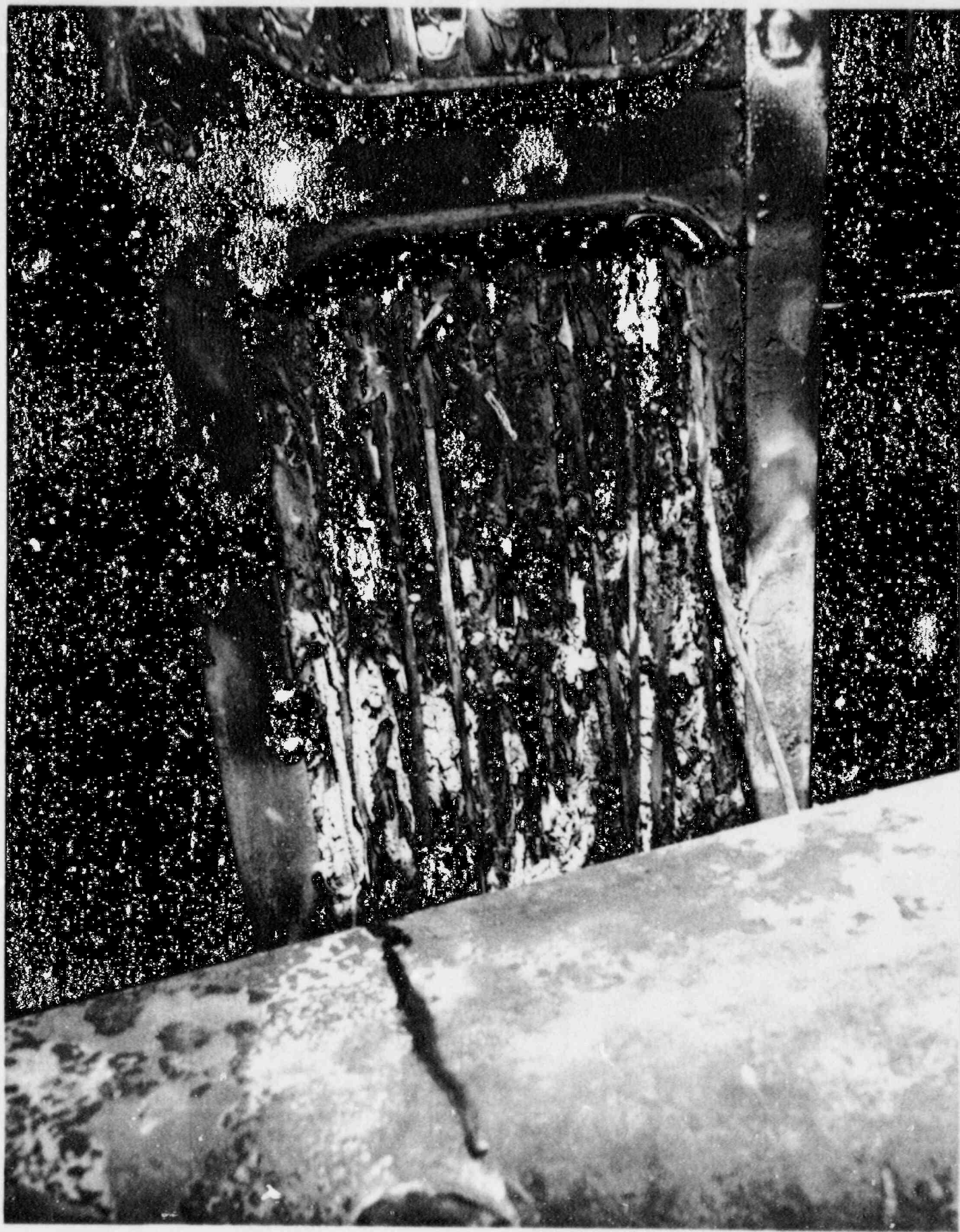
PICTURE NO. 16 Test No. 3 Cable Damage and Burner
