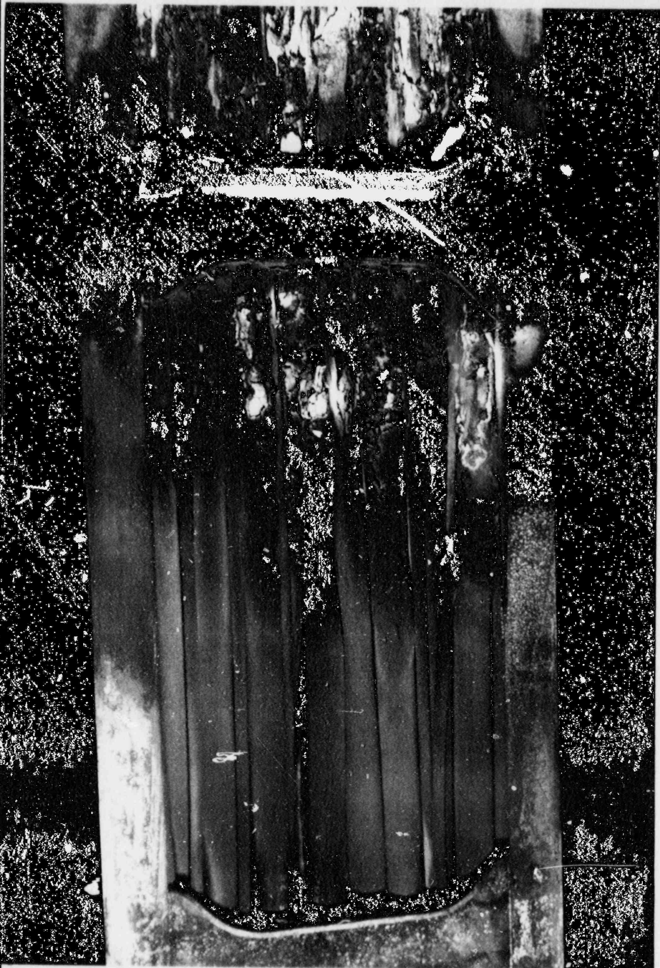
PICTURE NO. 14 Test No. 3 Cable Damage
