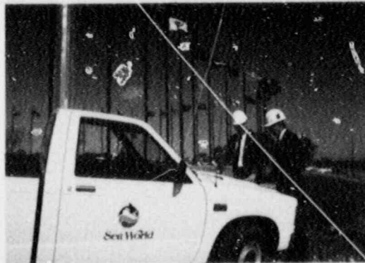
Sea World of Texas is expected to draw more than three million visitors in the park's first year of operation. Above, CPS Linemen help prepare the site for construction.
