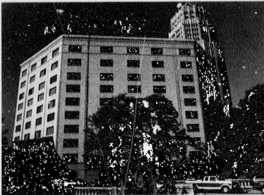
CPS' Main Office renovation added necessary office space for utility operation and attractive enhancement to the famed San Antonio Riverwalk.
