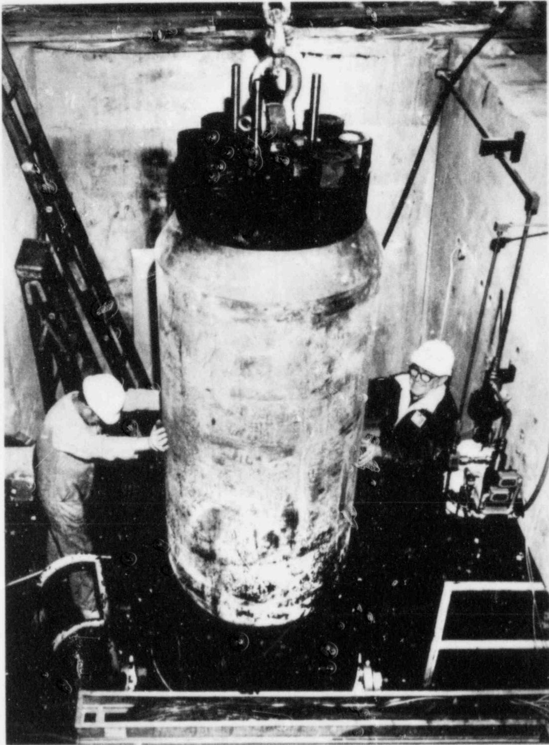
Fig. 10.2. Test vessel used for preliminary thermal hydraulic tests (PTSE-0) being lowered into shroud.
