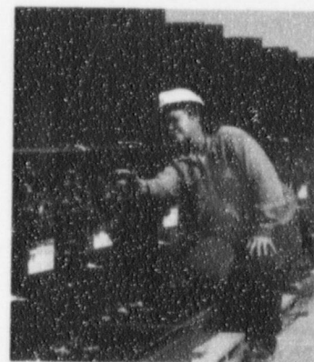
A warehouse employee inspects the padmount transformers which will be installed in neighborhoods with underground electric service.
