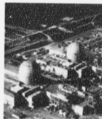
The South Texas Project, located on the Texas coast, was rated among the top producing nuclear plants in the country by the Nuclear Regulatory Commission.
