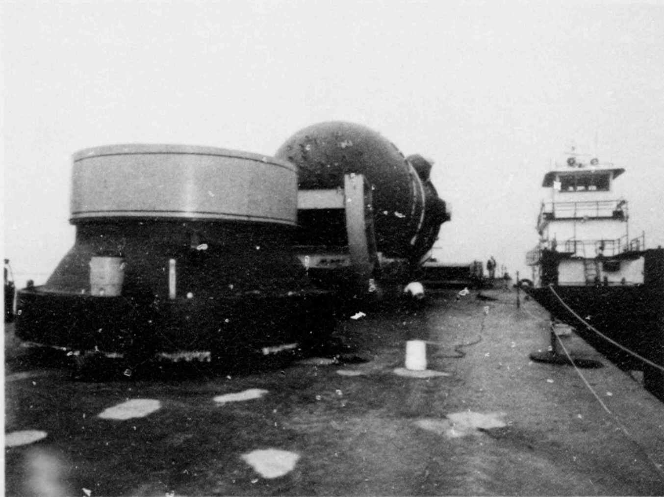
Fig. 11.6. View of PWR vessel and appurtenances loaded on barge at arrival at the K-25 barge slip.
