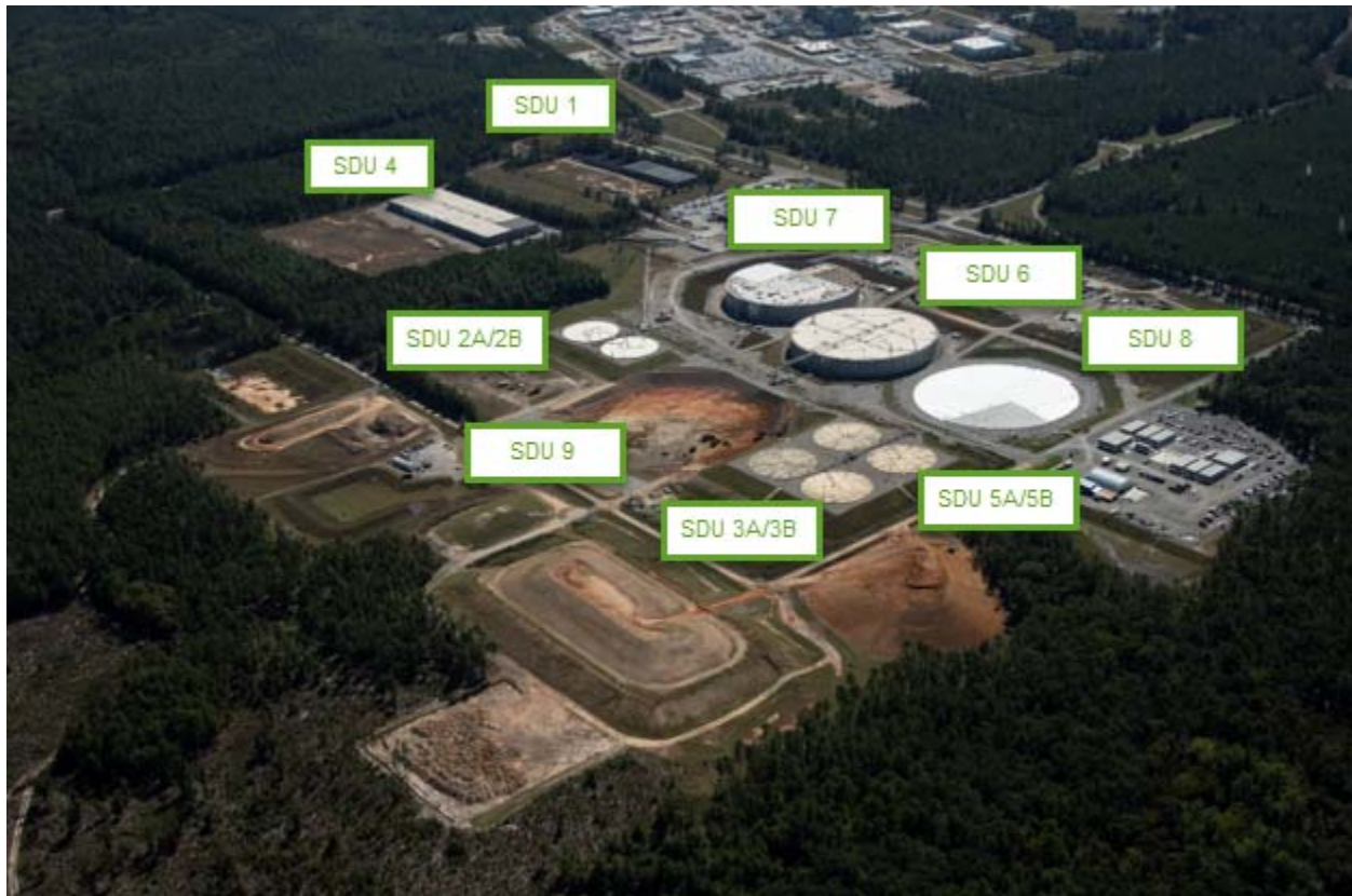
Figure 4.1-1: Saltstone Facility Aerial View (October 2019)
