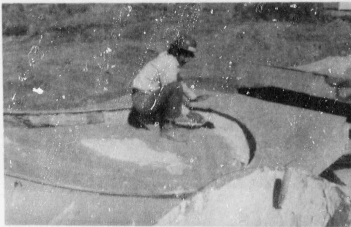
Figure 28. Fabrication of Wooden Form for the Equipment Hatch Boss.
