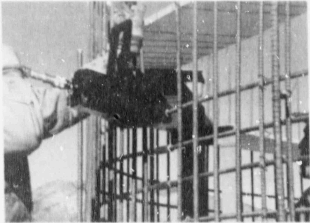
Figure 6. Swaging of Splices Using Hand-Held Press.
