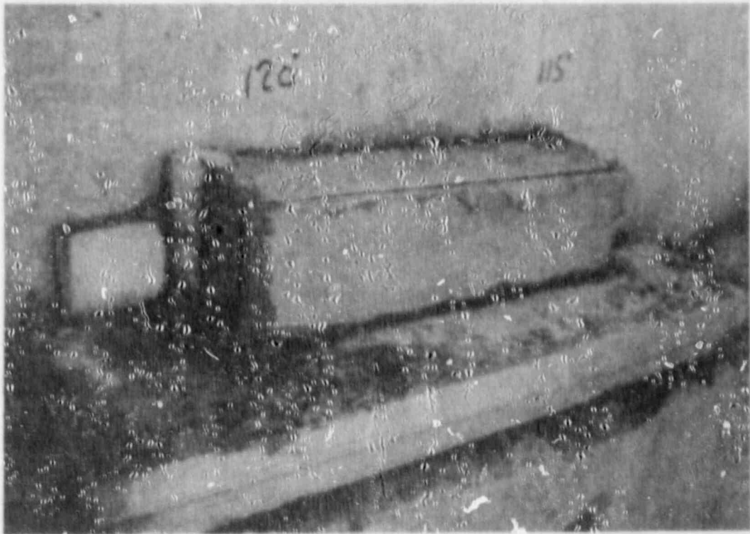
Figure 35. Repair Process of the Concrete Void in the First Cylinder Lift.
