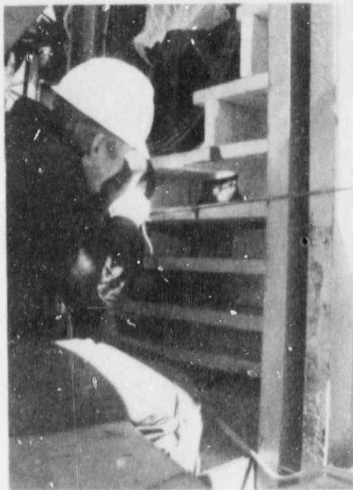
Figure 25. Placing of Concrete Around Boss 'A'.
