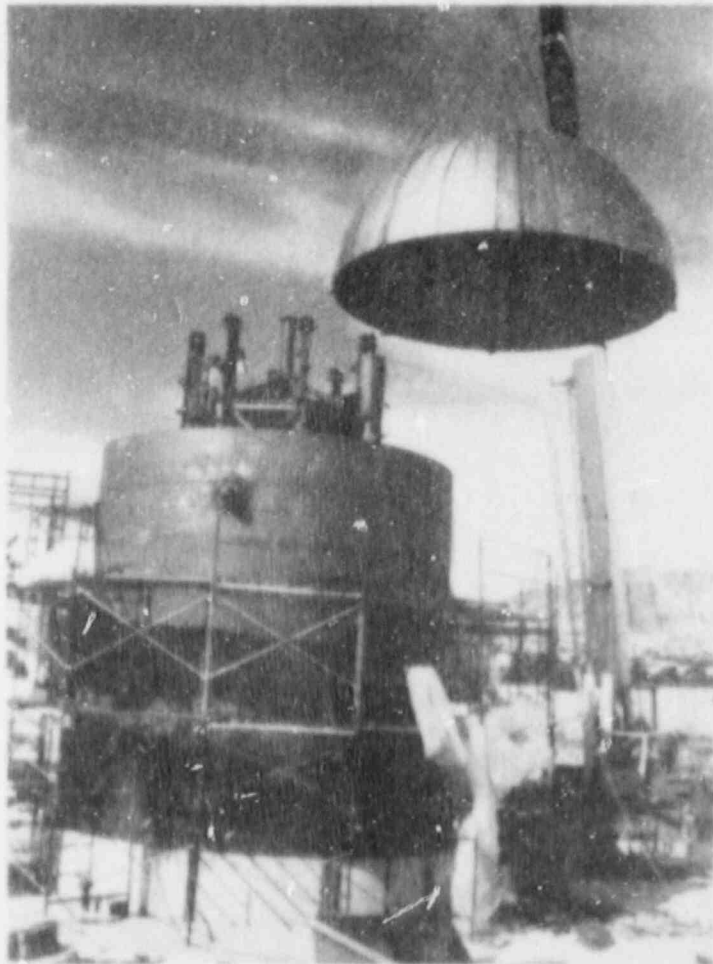
Figure 21. Placing the Dome Section of Liner on Cylinder Liner.
