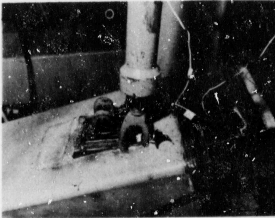
Figure 30. Broken eye of lower end of vertical strut from 8-in. butterfly valve test.
