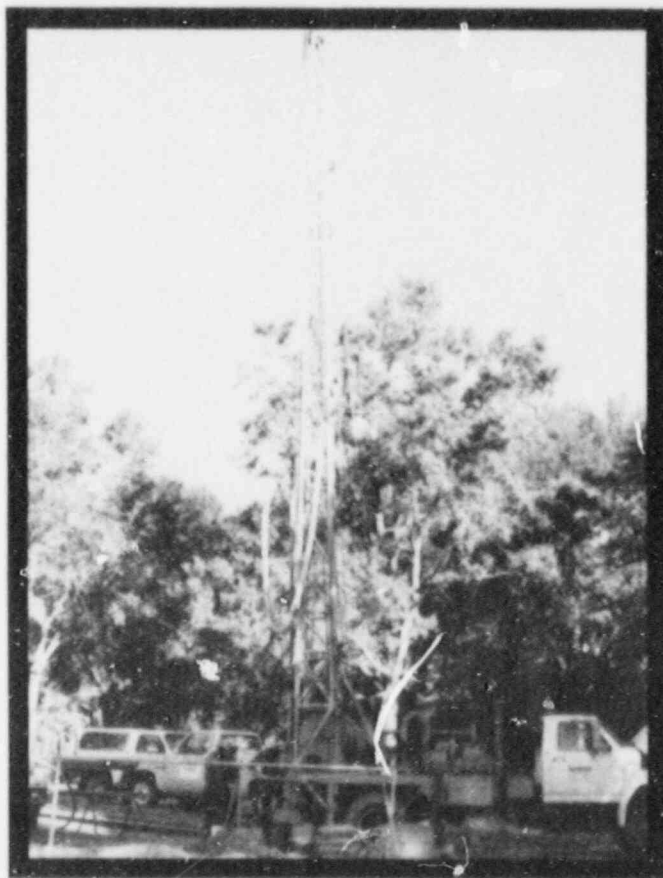
Thirty wells were installed in F Area in 1987
