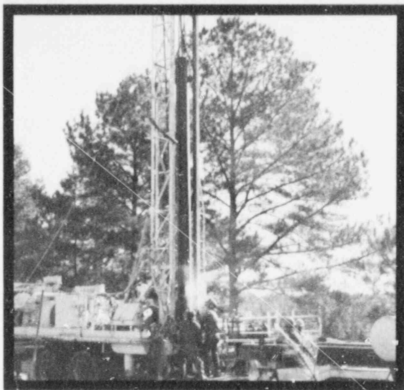
Installing surface casing for well
