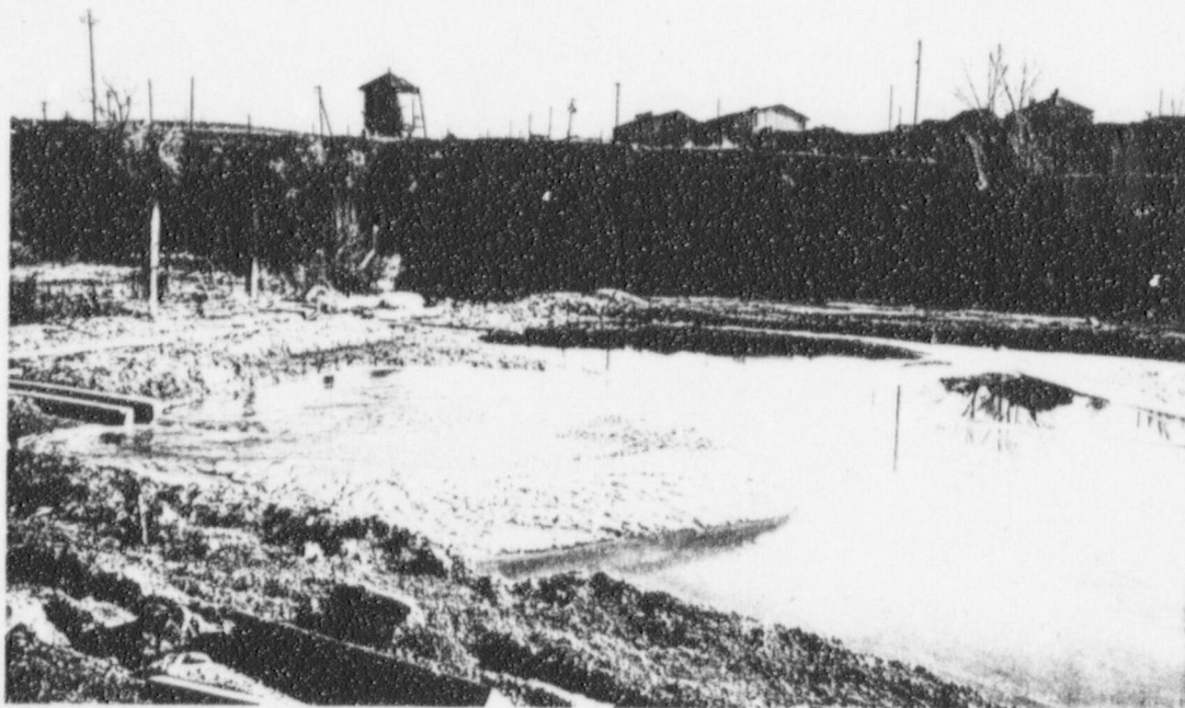
17. Settling pond for vanadium circuit effluent discharge.
