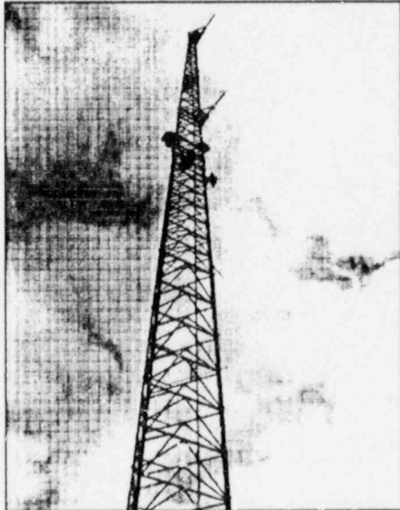
Fig. 1-10: Davis-Besse operates its own weather station. The main weather tower (shown here) is 100 meters tall and has 3 levels of sensors.
