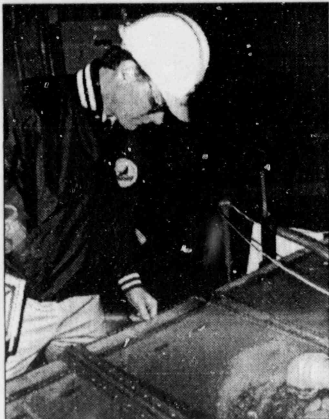
Fig 7-1: Clarified water is inspected prior to entering filters.
