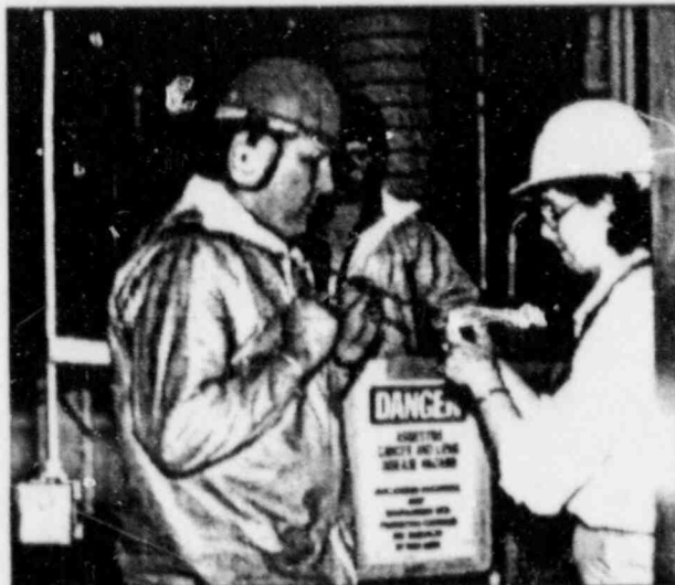
Fig. 8-4: A worker is fitted with a personal air monitor to measure fiber concentration during asbestos insulation removal.
