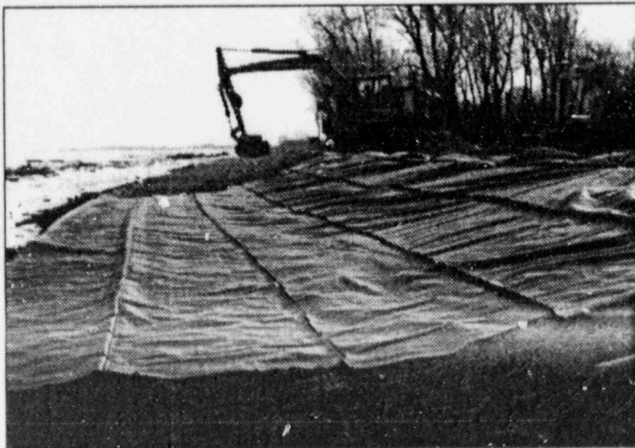
Fig. 6-10: Filter fabric is laid prior to stone to prevent loss of integrity to the revetment from wave action.
