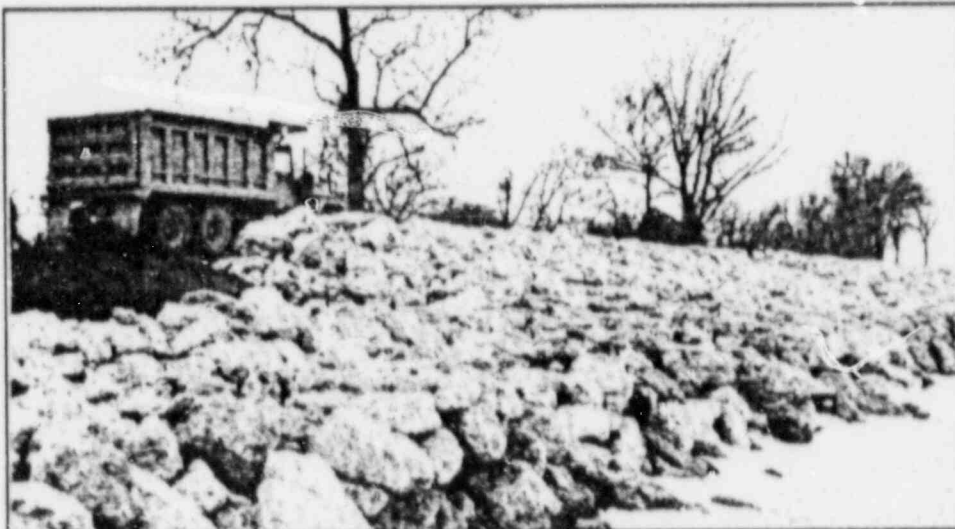
Fig. S-3: Davis-Besse continued to protect the marsh with the 1987 dike revetment construction project.
